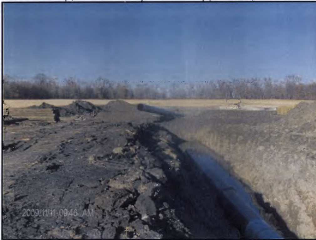
Restoring preconstruction contours of trenchline within wetland
