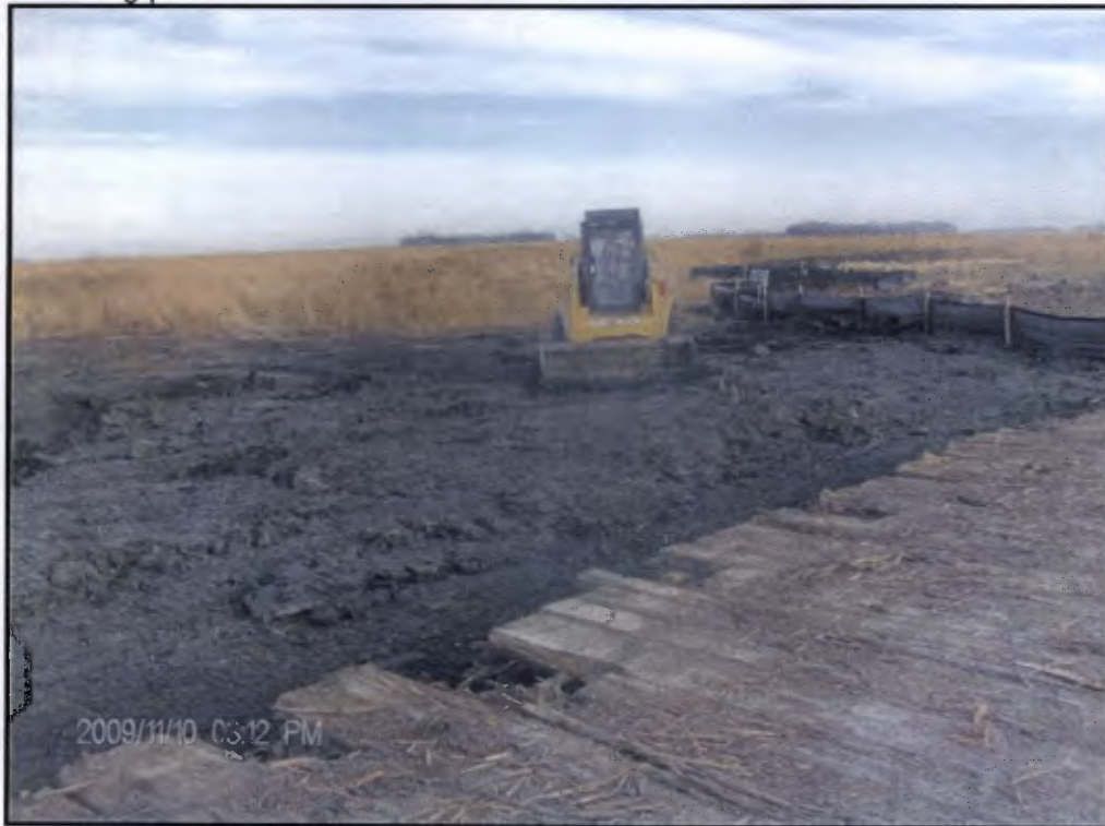
Restoring preconstruction contours of trenchline within wetland
