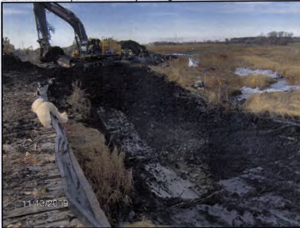
ECDs in place and functional at a wetland and waterbody crossing
