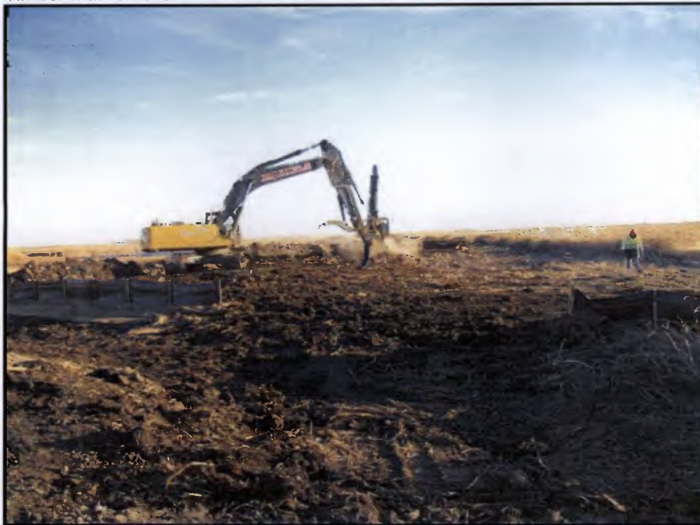
Timber mat removal
