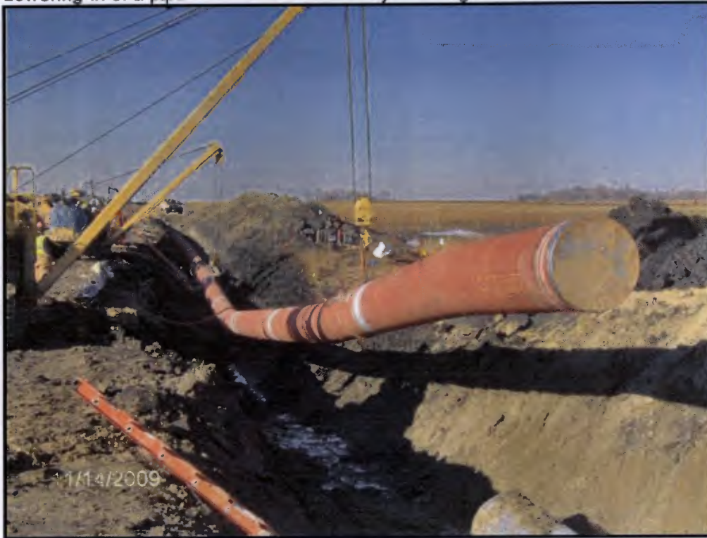
Lowering-in of a pipe section at a waterbody crossing
