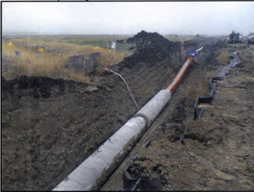
Tie-in on mainline section to Red River HDD pipe section
