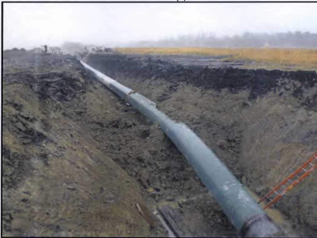
Tie-in on mainline section to Red River HDD pipe section
