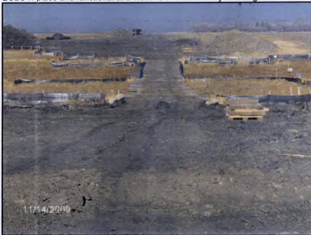
ECDs in place and functional at a wetland and waterbody crossing
