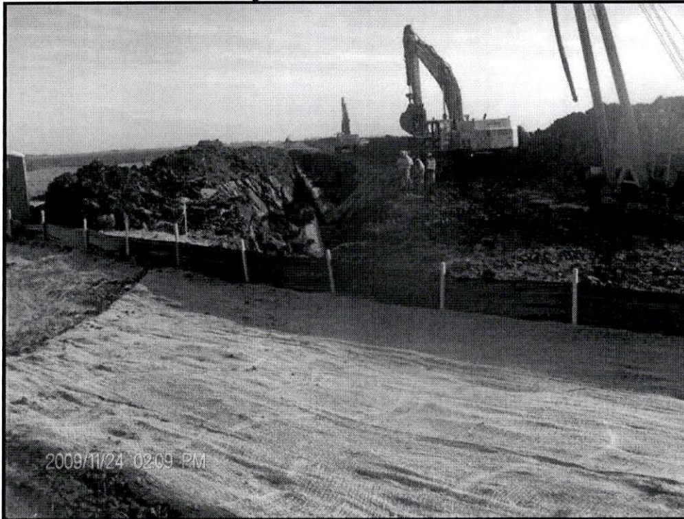
Tie-in location at road crossing
