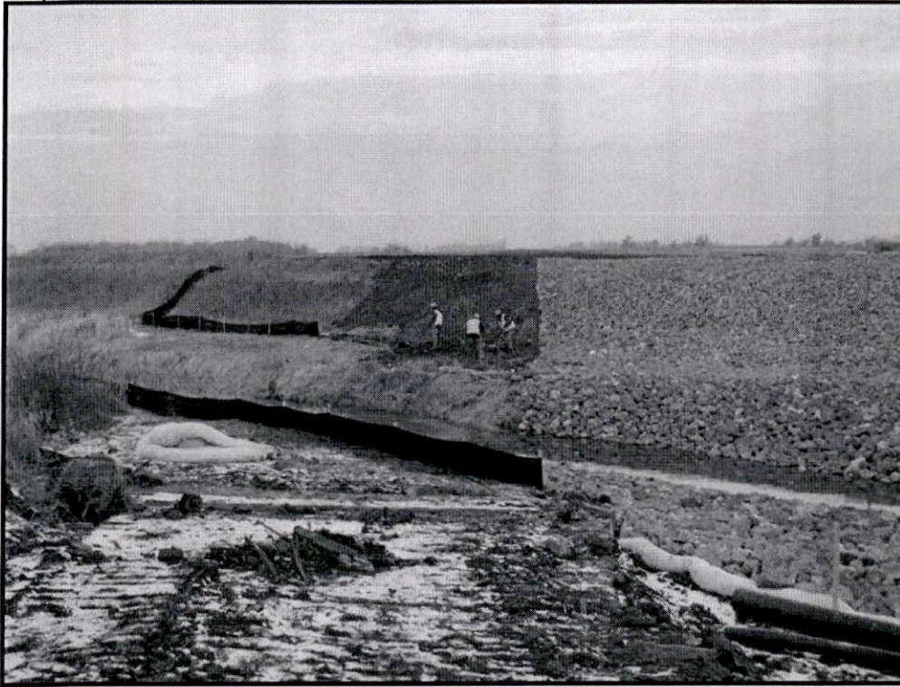
Topsoil stabilization
