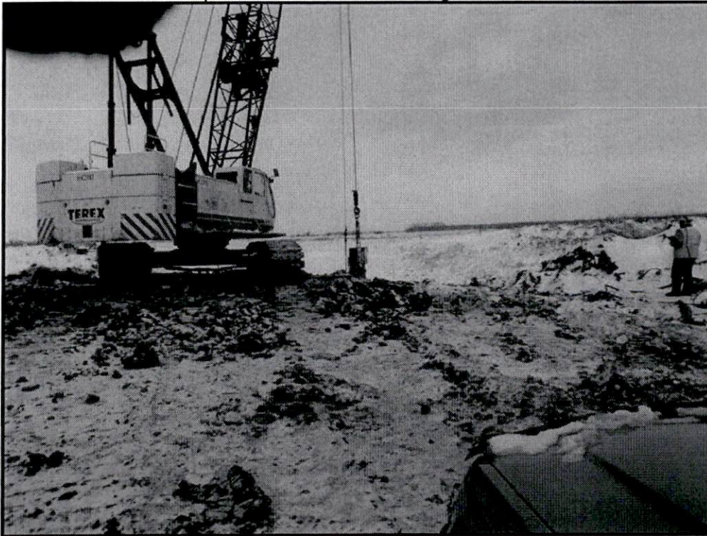
Removal of final sheet pile from south bank at Tongue River "Cutoff"
