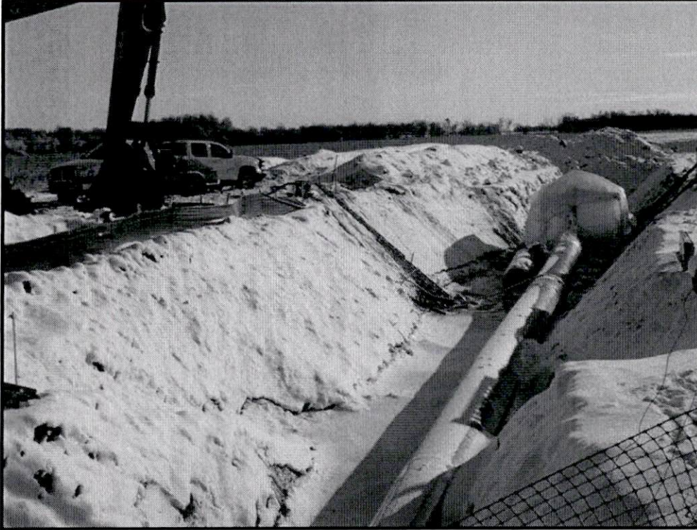
Removal of final sheet pile from south bank at Tongue River "Cutoff"
