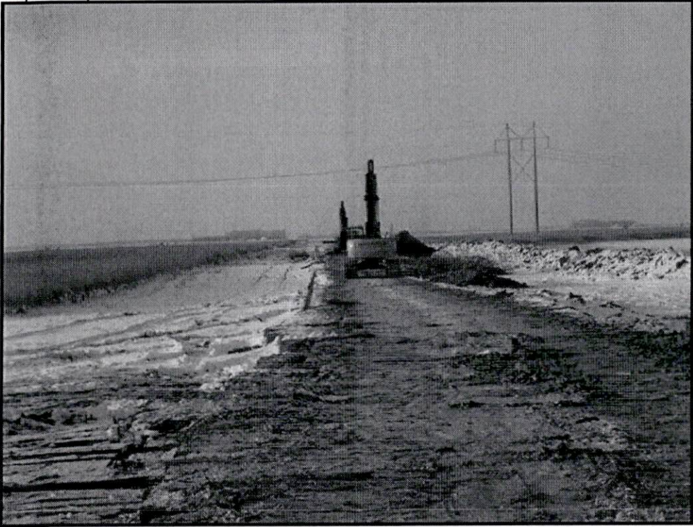
Topsoil replacement and timber mat removal within wetland w-791c
