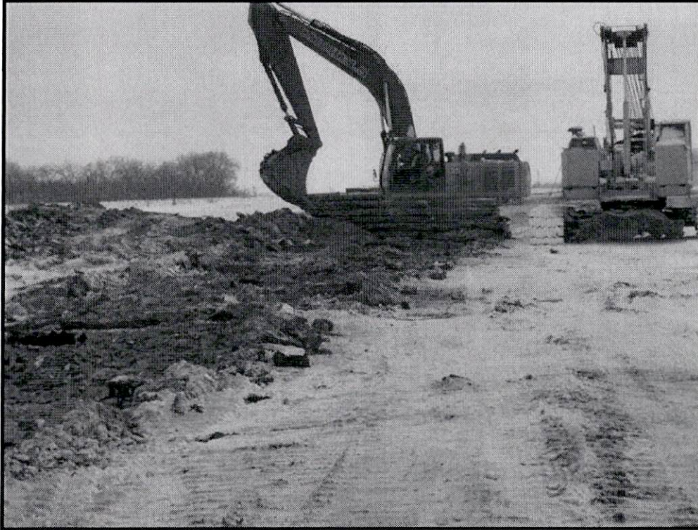
Timber mat removal and restoration at milepost 783.4
