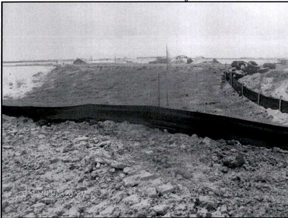
Erosion Control Devices Installed at a Ditch Crossing
