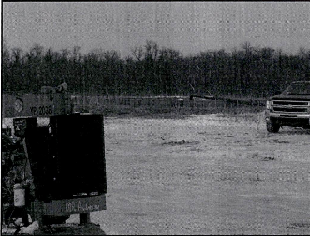
Hydrostatic Test Dewatering Filtration and Energy Dissipation Structure
