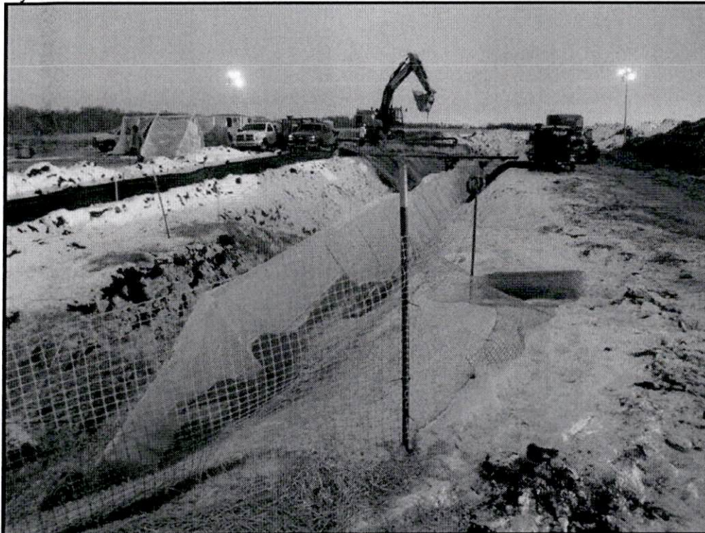
Hydrostatic Test Location near Red River
