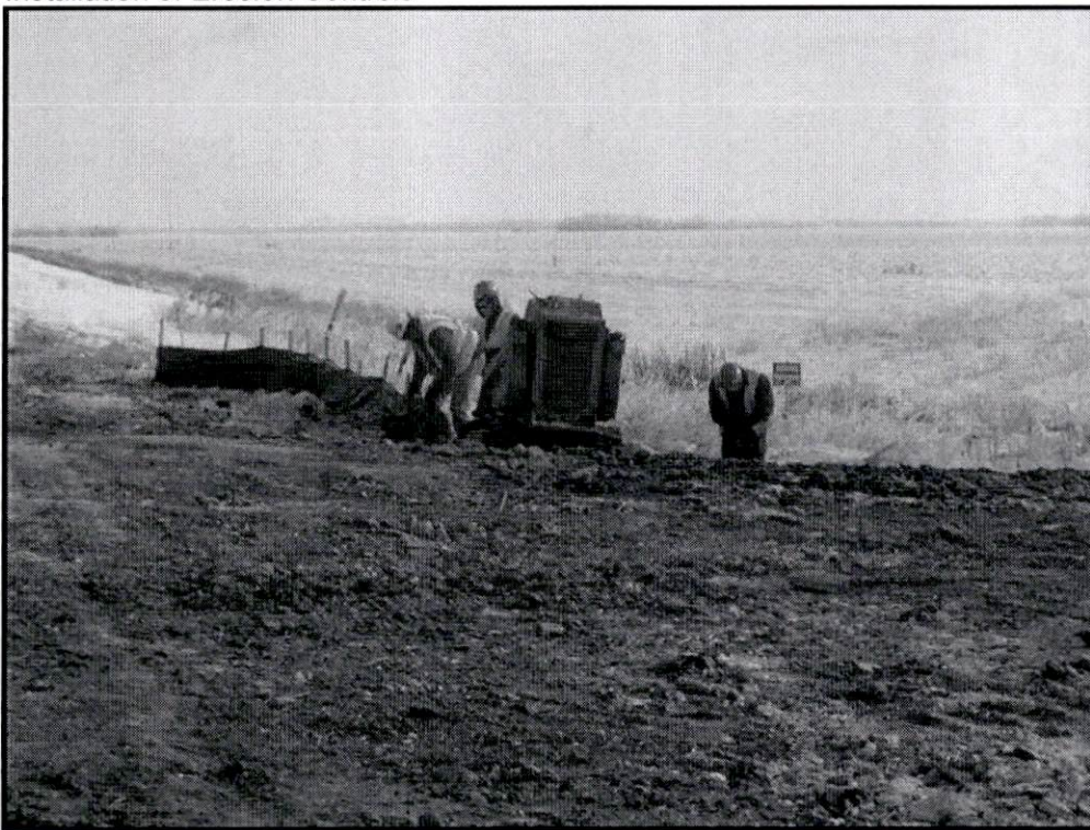
Installation of Erosion Controls
