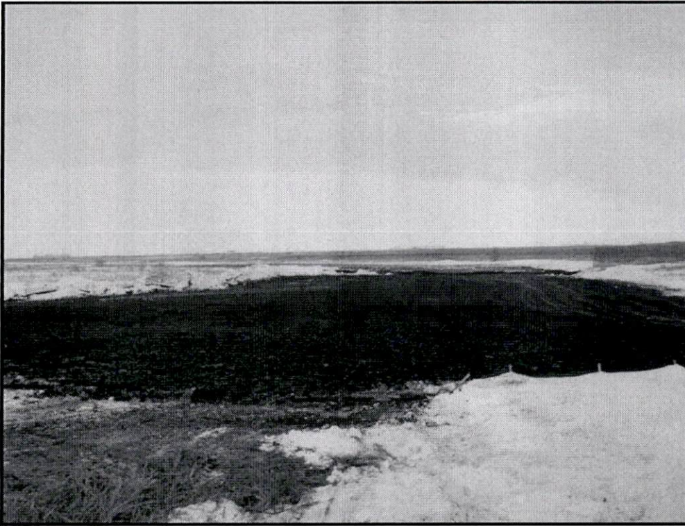
Mulching of Right-of-way Adjacent to Wetlands
