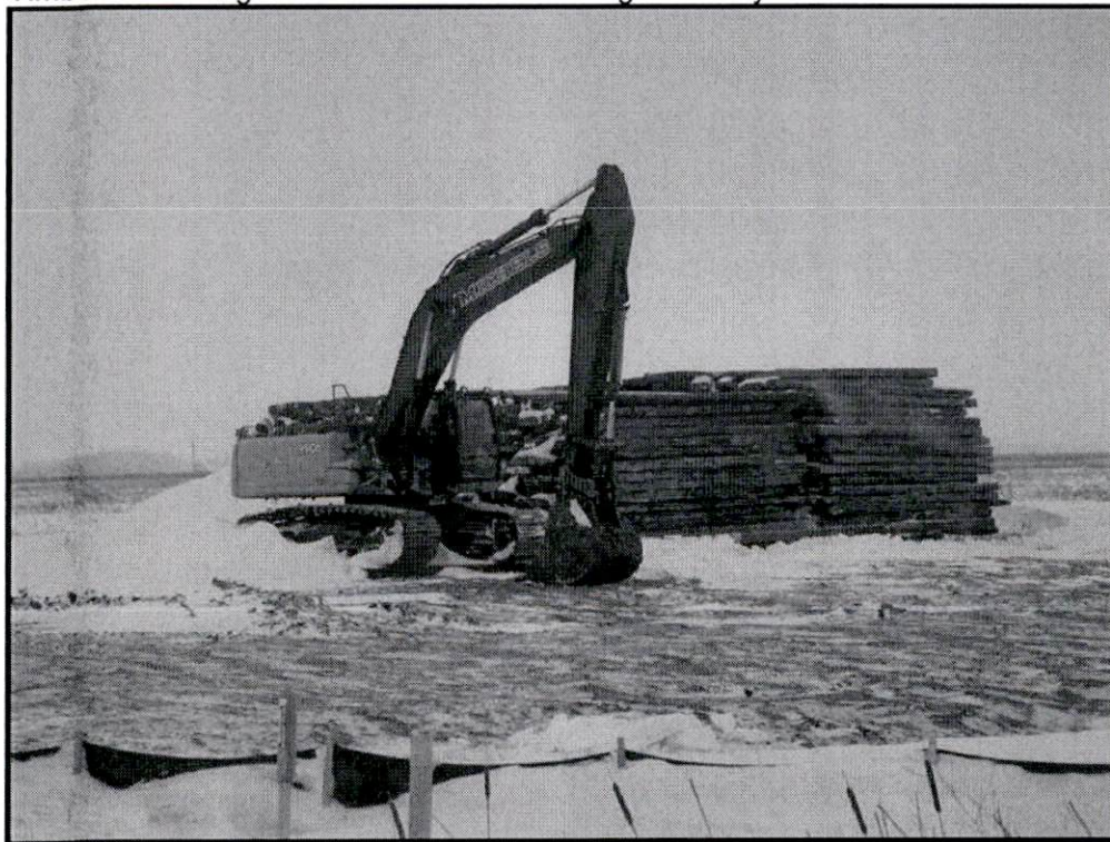
Timber Mats Staged for Removal from the Right-of-Way
