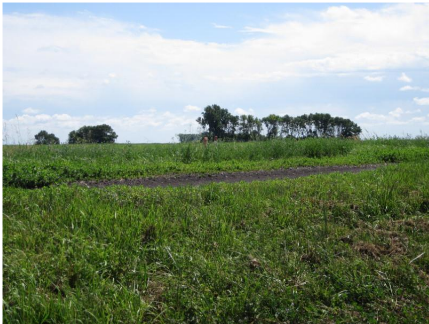
Photo 34. Direction: Southeast. Looking across a minimum maintenance portion of 154 th Ave NE at Mile 787 with ditch in the foreground and field in the distance. Crops, soils, and ditch vegetation were in good condition. The road had a slight depression from being open cut along the pipeline route.
