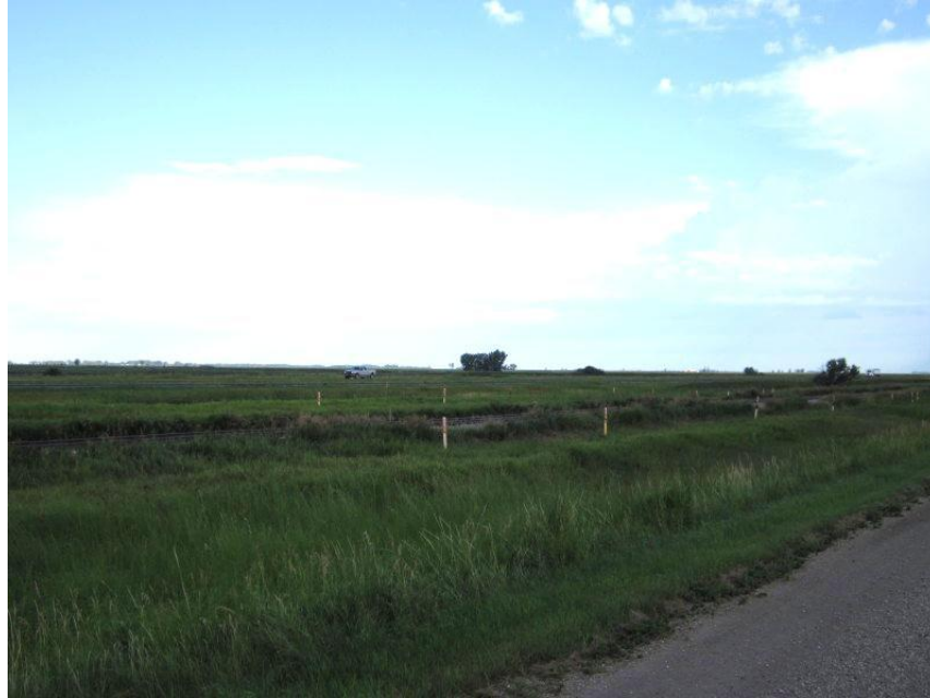
Photo 1. Direction: Northwest. Pipeline markers from left of photo denote Alberta Clipper and LSR pipelines to the east of Mile 795 of the pipeline route. Interstate 29 in the distance (on which pickup is located), Burlington Northern Railroad in mid-ground, the gravel frontage road in foreground, and a wetland on the west side of Interstate 29 (not visible) were all crossed underneath using one large horizontal drilling bore to avoid impacts to all these features. The railroad was cultural site 32PB0173.
