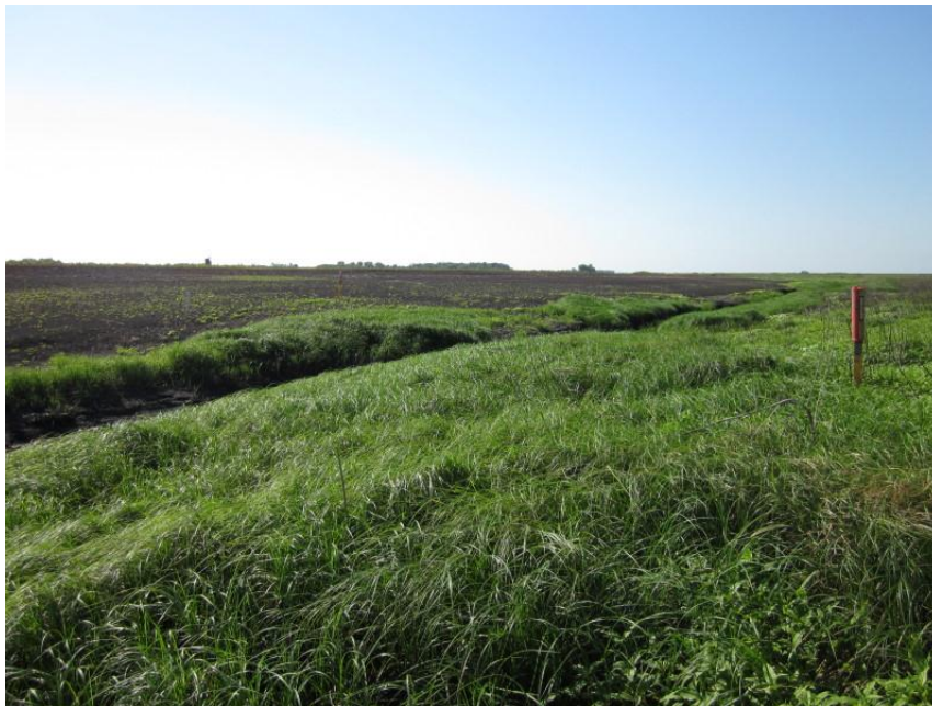
Photo 14. Direction: South. View of County Ditch 66-1 to the south, which diverges from the Red River within 0.5 miles north of this point. The crossing of the pipeline is indicated by the marker posts on either bank, and is just to the northwest of Mile 801. This crossing was directionally drilled underneath the ditch. There were no indications of vegetation disturbance or erosion problems.
