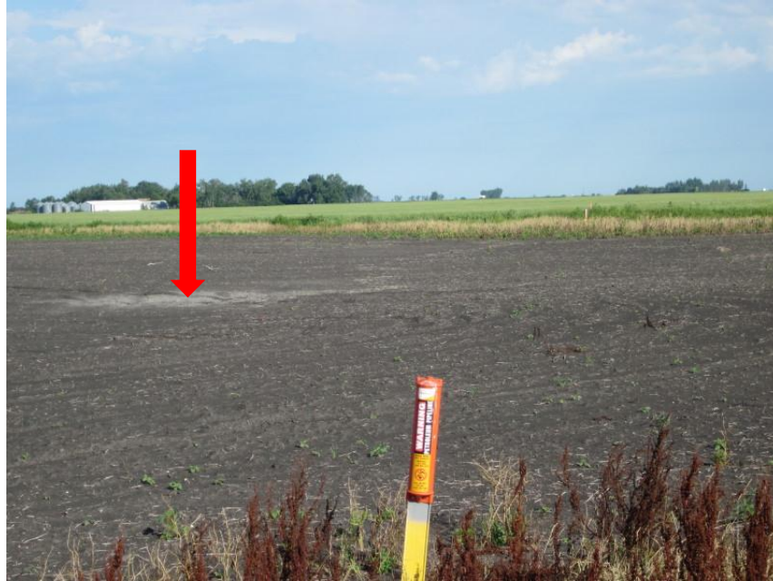
Photo 9. Direction: Northwest. View of field to the northwest of crossing of 161 st Ave NE. There was a depression in the field within the construction right-of-way but off the pipeline route which may be due to settling or improper topsoil replacement (red arrow), though it may also be a natural depression. Pipeline markers were in place along 161 st Ave NE (foreground).
