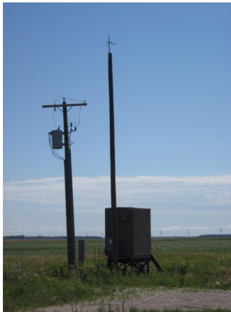
Photo 24. Direction: Southeast. Densitometer next to the valve system, which measures the density of the oil flowing through the pipeline. Information on the line served was not available at the time of the survey.
