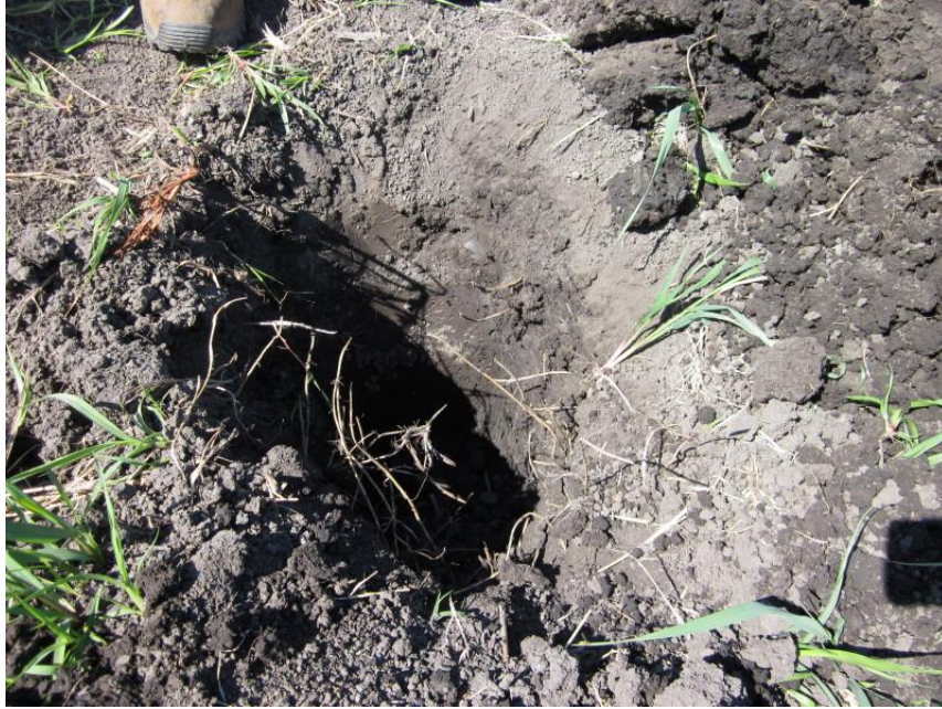
Photo 17. Topsoil exploration pit in an agricultural field north of 109 th St NE within the pipeline right-of-way (at approximately Mile 774.5). Topsoil went to a depth of greater than 20-inches. Subsoil could not be distinguished.
