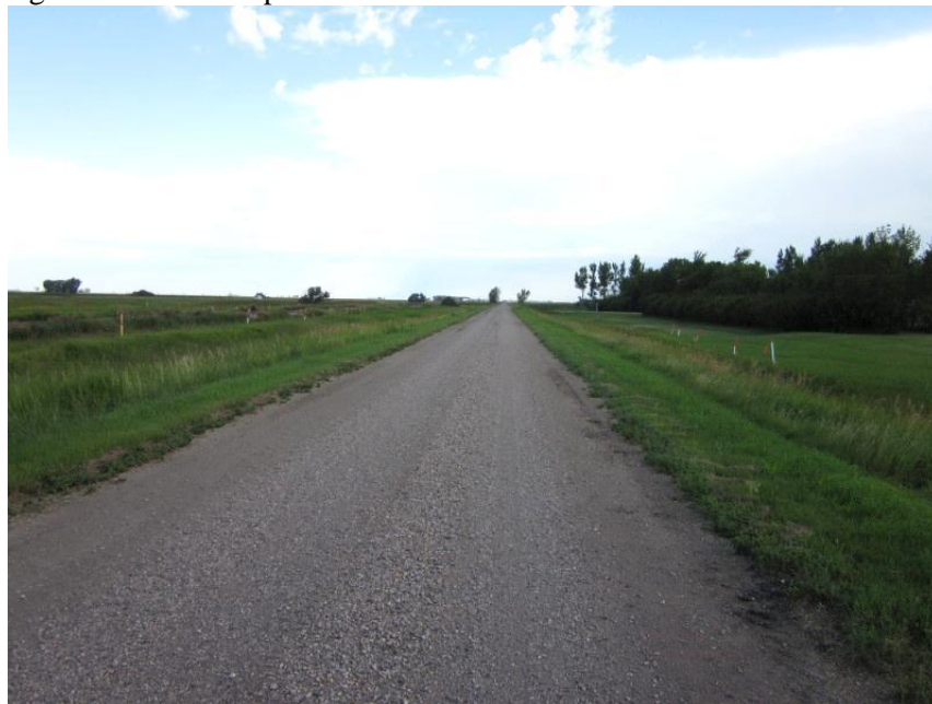
Photo 2. Direction: Northwest. Frontage road (Old Highway 44) to the east of Interstate 29 crossed underneath by the pipelines. All markers were in place and it appeared no vegetation had been disturbed in the ditches.
