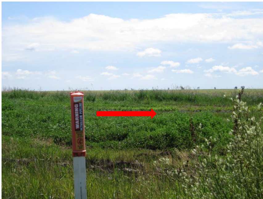
Photo 36. Direction: Southeast. Crossing of minimum maintenance 98 th St SE at approximately Mile 789.5. The crops and road ditches were in good condition but there was a slight depression in the road bed where the open cut had crossed (red arrow) which should be monitored.
