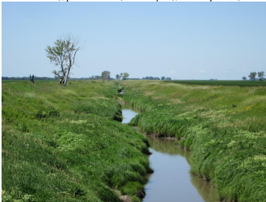
Photo 32. Direction: West. Tongue River cutoff ditch which had been open cut. The crossing of the pipeline is in the distance (though markers are not visible on photo). There were no revegetation or erosion problems.
