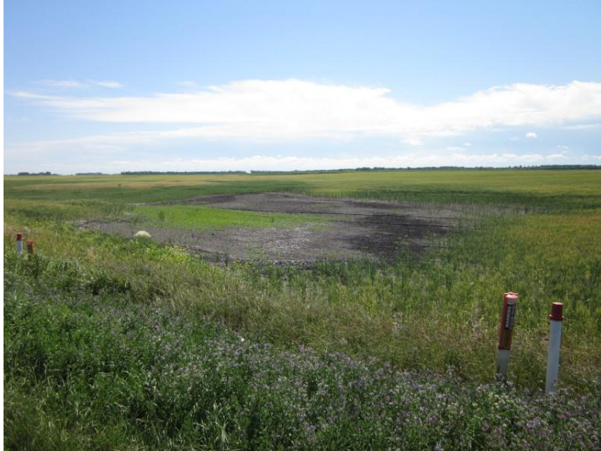
Photo 33. Direction: Southeast. Field southeast of 102 nd St NE at Mile 784 had a restored wetland depression (based on aerial imagery) within the pipeline route. Road had been bored underneath and all markers were in place.
