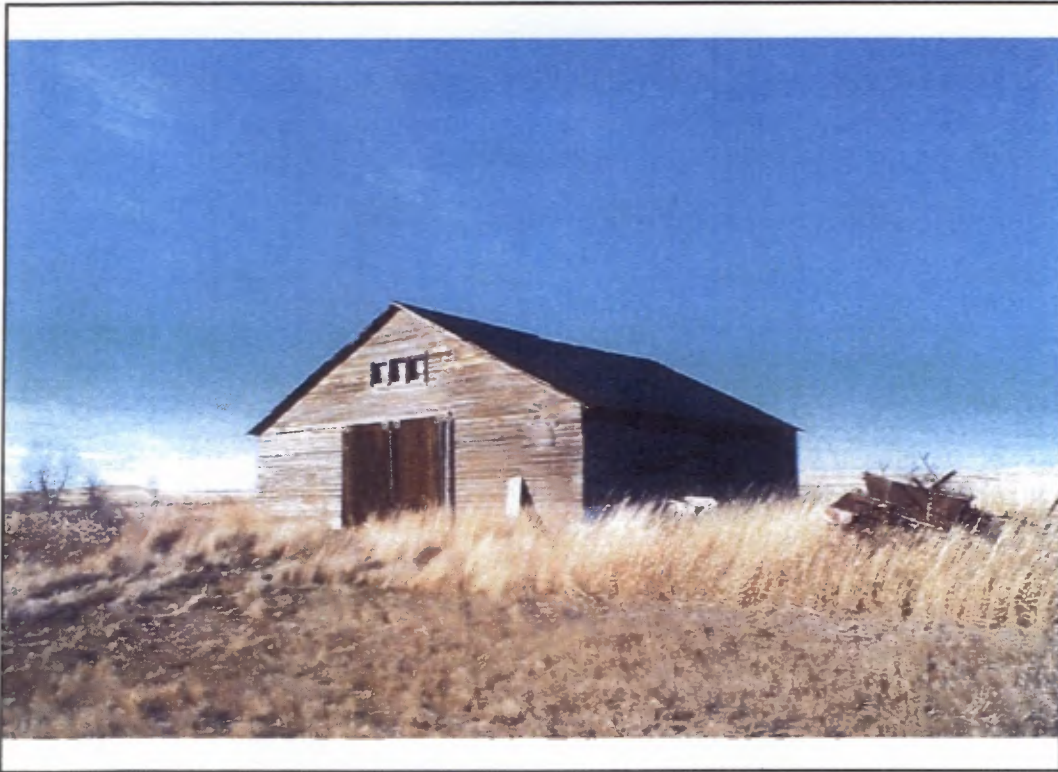
Figure 10 View of F2 on 32BO339 looking to the northwest. A concrete foundation (F4) is immediately to the right, but obscured by the high grass.
