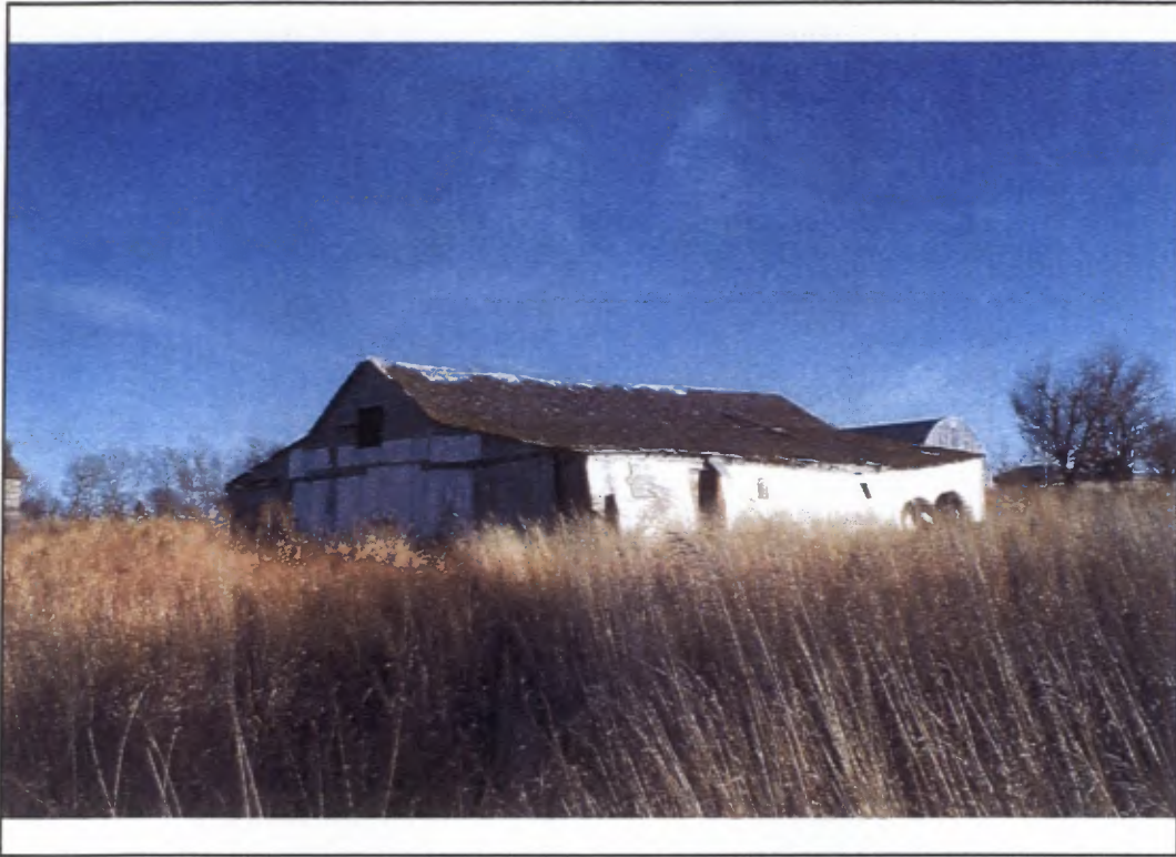
Figure 11 View of F3 on 32BO339 looking southeast. The modern Quonset building is just visible over the right corner of F3.
