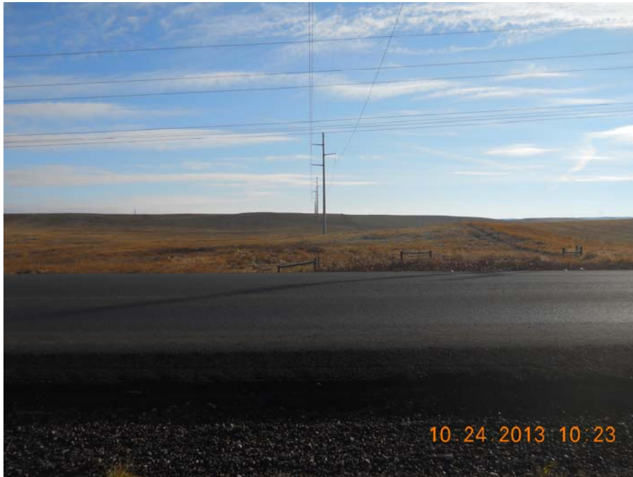
Photo 14 – Direction: East – Transmission line at road crossing directly north of Rhame Substation.
