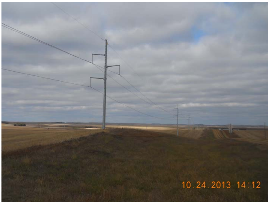
Photo 27 – Direction: North – Transmission line parallel to county road on edge of cropland. Notice complete reclamation.
