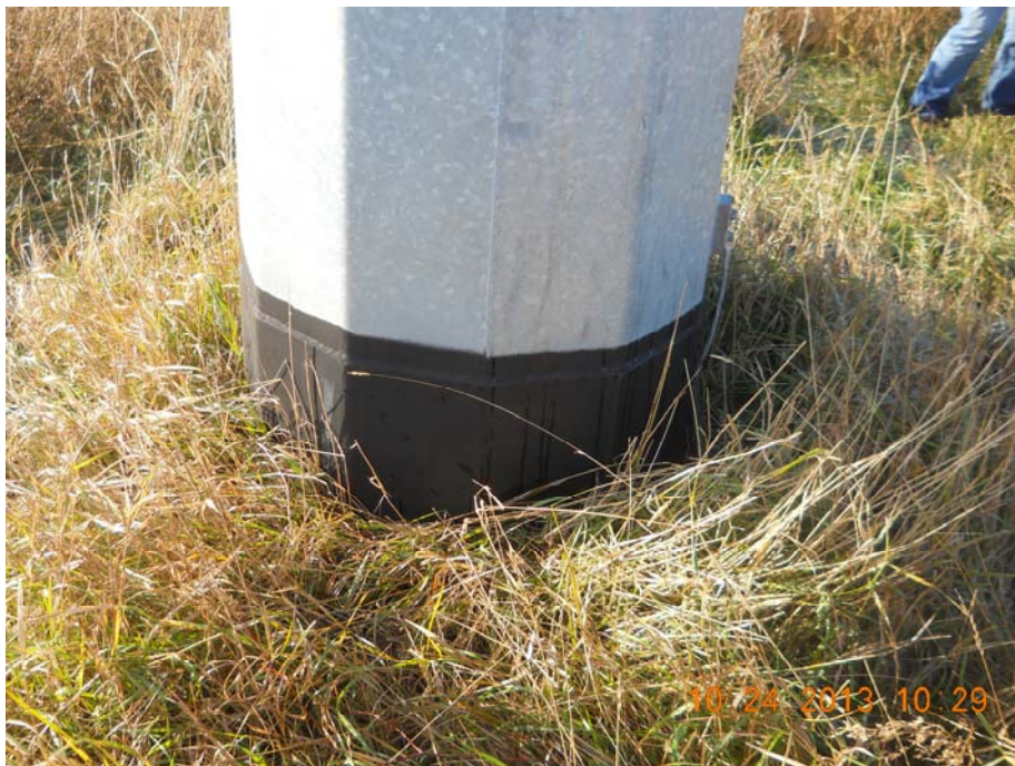
Photo 15 – Showing base of standard structure.
