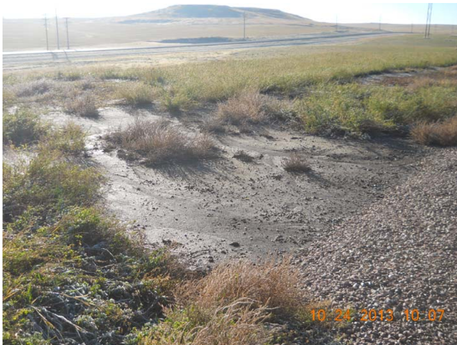
Photo 13 – Direction: Southeast – Closer photo showing vegetative die-off noted in Photo 12.
