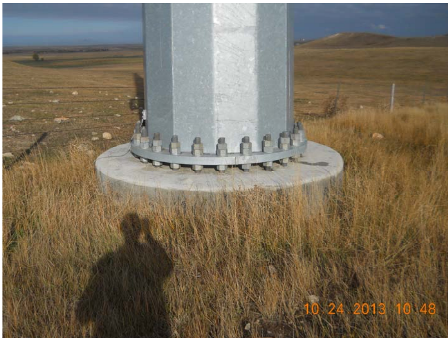
Photo 17 – Showing foundation and base of angle structure.
