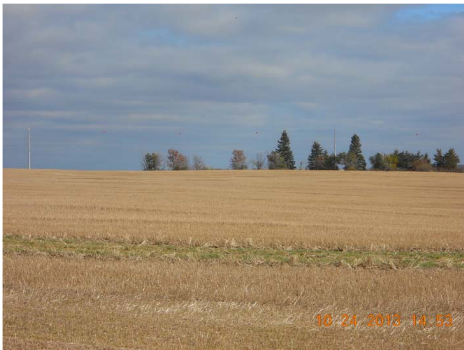
Photo 32 – Direction: East – Bird flight diverters in place on transmission line approximately 16 miles southeast of Belfield, ND.
