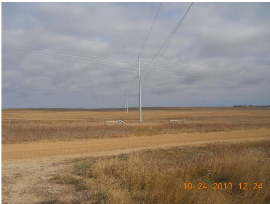
Photo 23 – Direction: Northeast – Transmission line moving northeast. Notice the completed reclamation and fence and gates in good condition.
