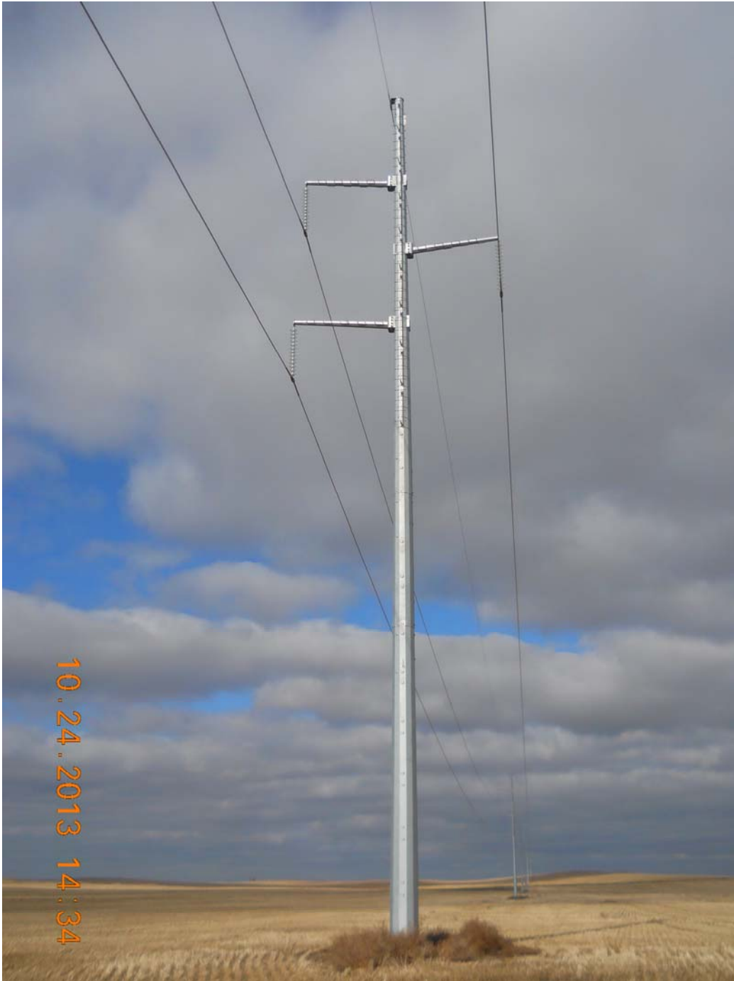
Photo 30 – Direction: North – Same location at Photo 29. Showing minimal loss of cropland around base of structure.
