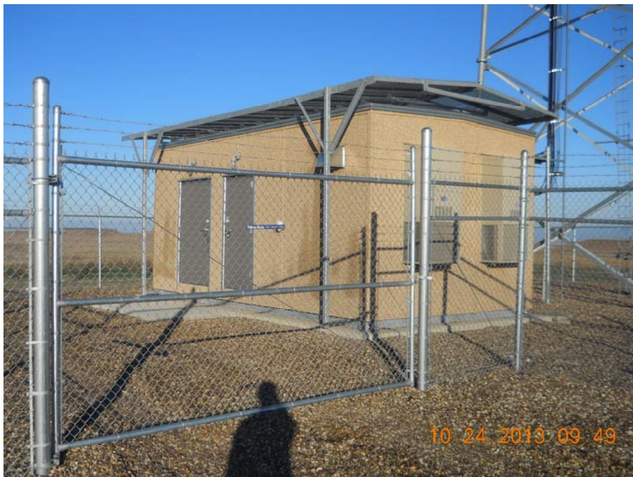
Photo 6 – Direction: West – Utility Building associated with the Rhame Microwave Tower.
