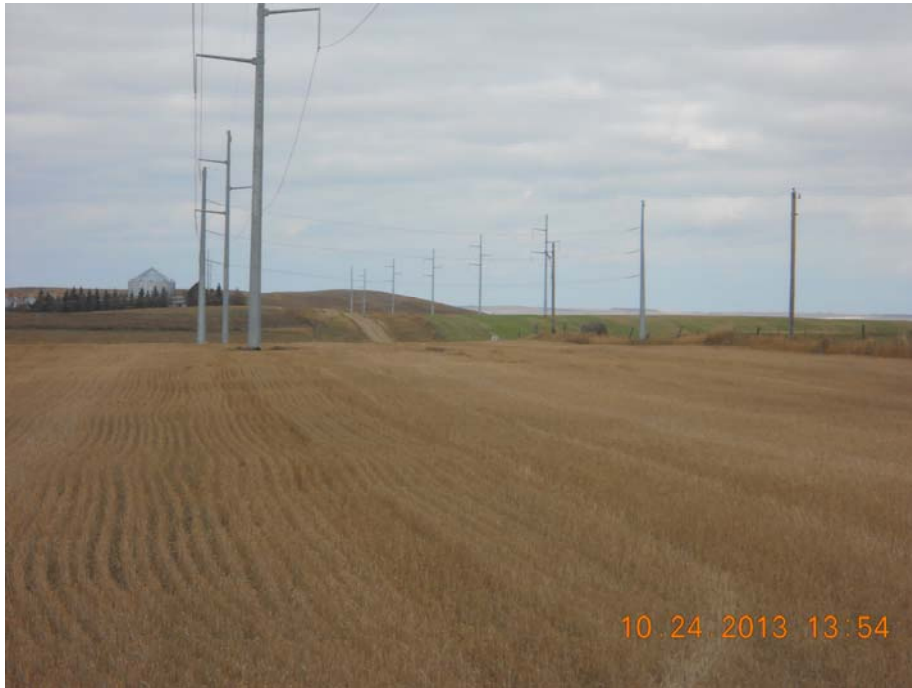
Photo 26 – Direction: North – Showing transmission line crossing county road directly north of ND 21 to avoid a farmyard.
