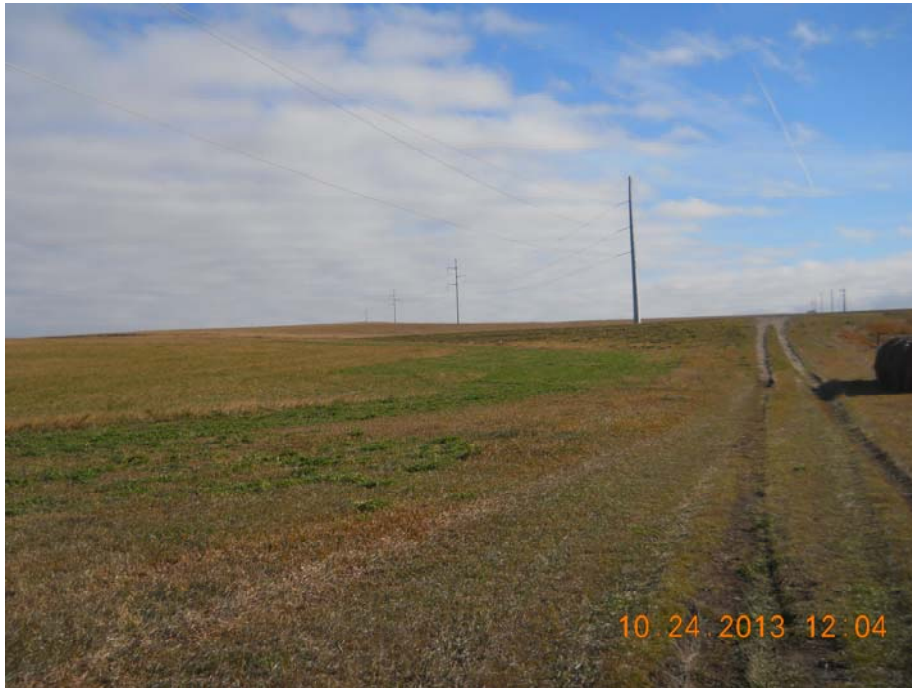
Photo 21 – Direction: East – From west side of US 85. Showing road crossing and angle structure where line moves northeast.
