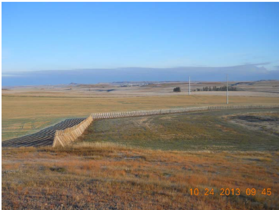
Photo 4 – Direction: North – Showing shield fence to the north/northwest of Rhame Substation.
