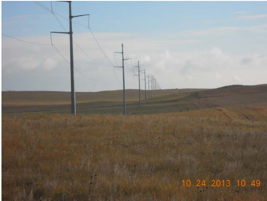
Photo 18 – Direction: East – Showing complete reclamation along the transmission line.
