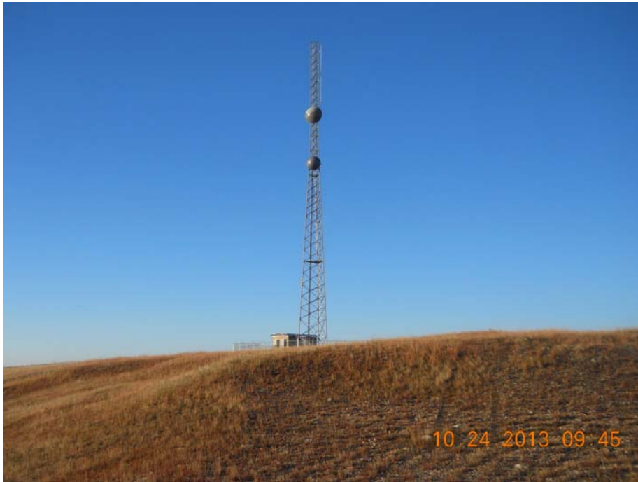
Photo 5 – Direction: Southwest – Rhame Microwave Tower.
