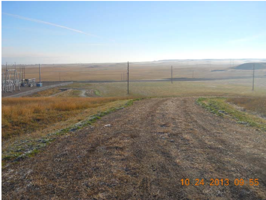
Photo 7 – Direction: East – Access road to Rhame Microwave Tower from Rhame Substation.
