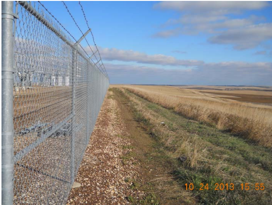
Photo 37 – Direction: East – Well maintained gravel perimeter and fence at Belfield Substation.
