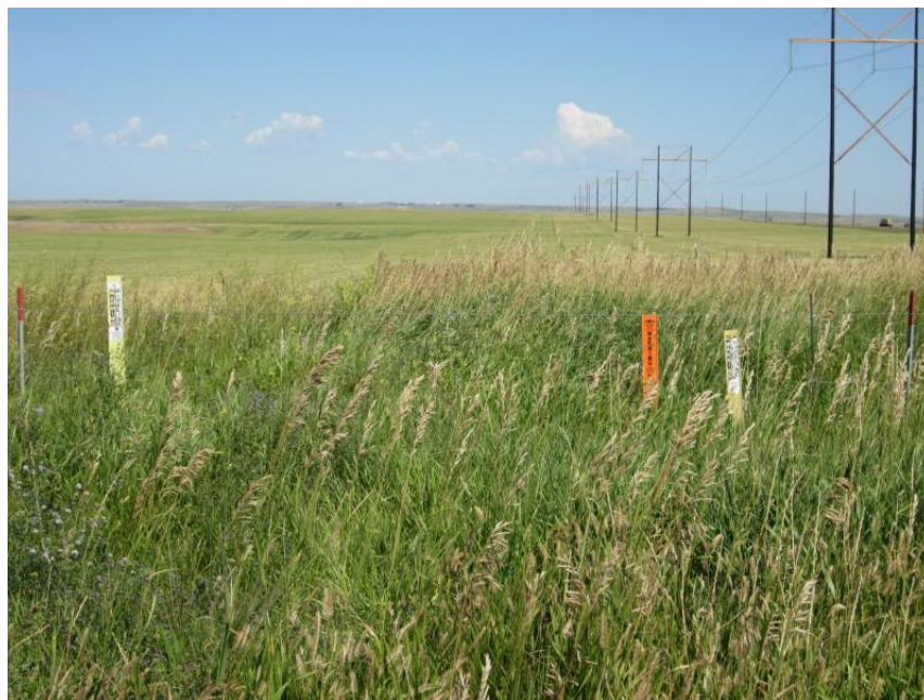
Photo 10. Direction: North. View of cropland in good condition in the SE ¼ of the SE ¼ of Section 19, T151N, R101W. Pipeline markers are in the ditch of Highway 200 and indicate the horizontal drill used to cross the road, which runs east-west between Sections 19 and 20. The ditch vegetation had good cover except for a few insignificant bare spots.
