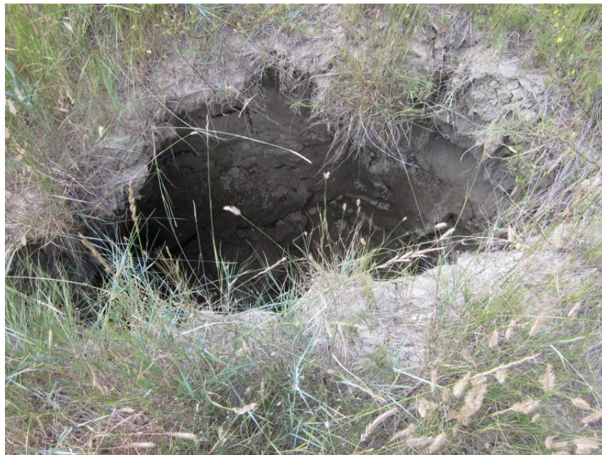
Photo 30. Close-up of a hole to a depth of 5 to 6 feet within pipeline right-of-way leading up to the north edge of another tributary drainage of Spring Creek in the SE \frac{1}{4} of the SE \frac{1}{4} of Section 27, T148N, R102W. The hole was likely caused by piping of water, in which flow is concentrated along the buried pipeline and begins to erode the recently reclaimed loose soils, eventually reaching the surface and forming a hole.
