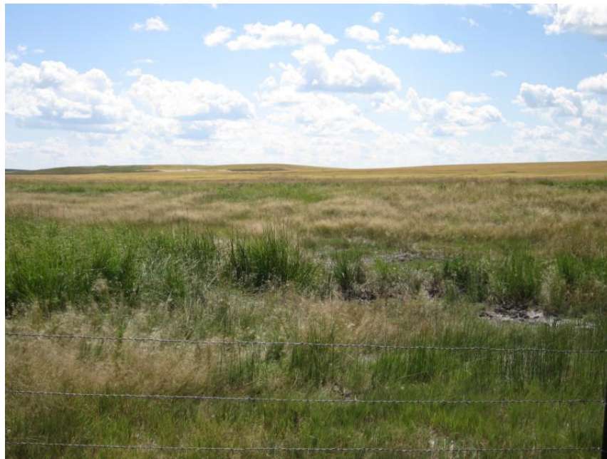
Photo 18. Direction: South. Pipeline crossing of Antelope Creek in the NE ¼ of Section 31, T150N, R101W. As-builts indicated this crossing was open cut. Revegetation of the creek appeared satisfactory. Native plants had colonized the right-of-way including prairie cordgrass ( Spartina pectinata ), Nuttall's alkali grass ( Puccinellia nuttalliana ), and dock ( Rumex sp.). There were no trees or shrubs along the creek. The cropland to the south appeared to be in good condition. Note the fenceline in the foreground which was new and had been replaced after pipeline construction. Markers were not present.
