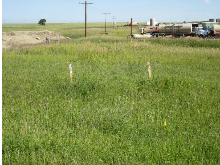
Photo 1. Direction: North. North end of pipeline route (denoted by yellow markers in ditch) looking toward oil service facility, which the pipeline tied into at the south end of the SW ¼ of Section 18, T152N, R101W, McKenzie County, ND.
