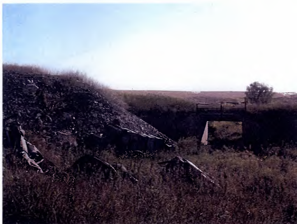
Figure 85: View east over dump and bridge, site 32WI1008 (Image #737).
