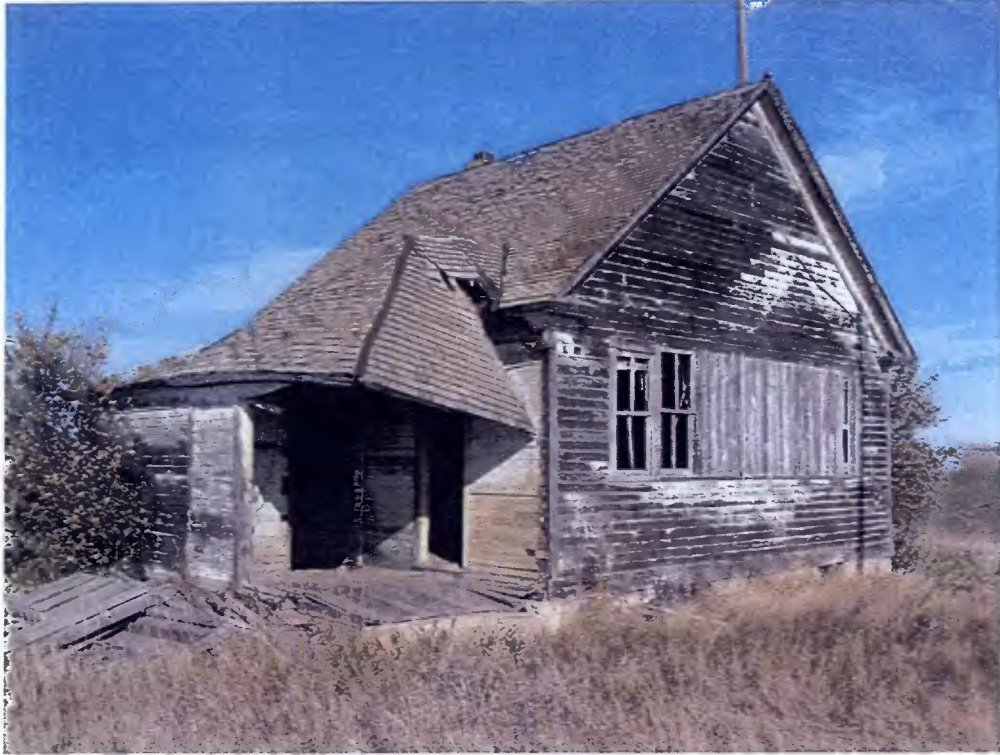
Figure 110: View northwest over school site 32W11033 (Image #816).
