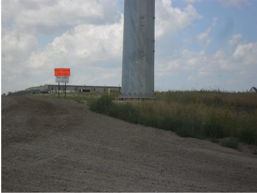
Photo 9 - Showing foundation and base of an angle structure
