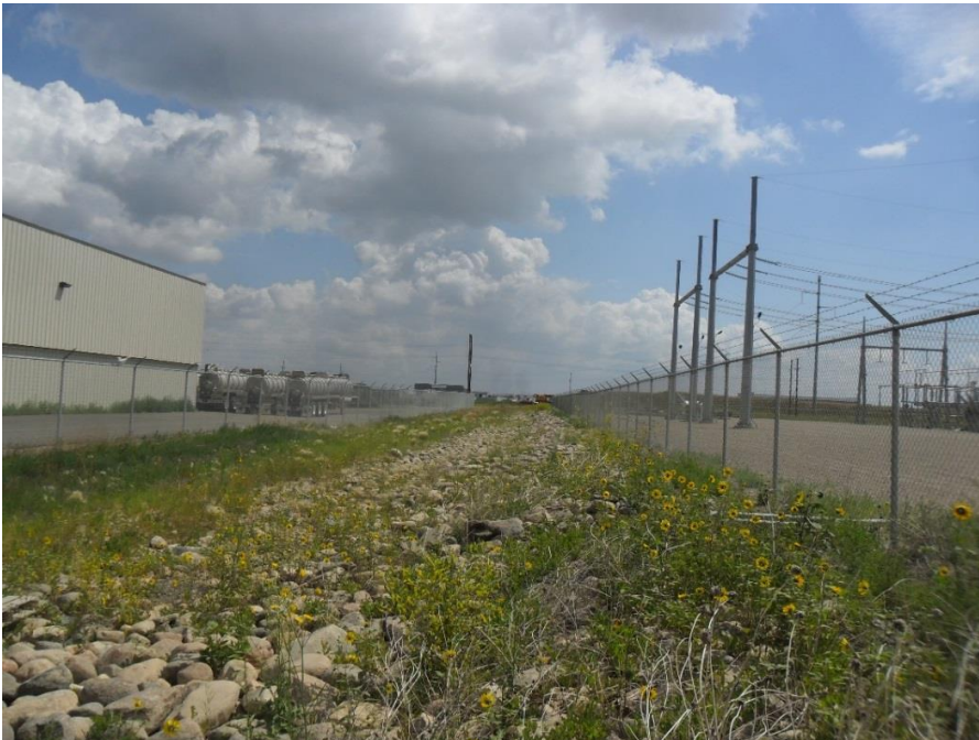
Photo 4 - Direction: East - Showing weeds on North side of Williston substation.
