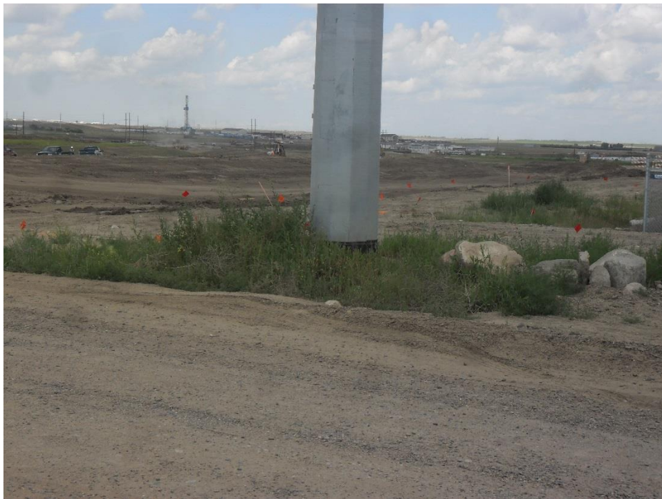
Photo 8 - Showing base of structure.
