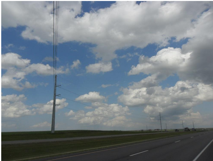
Photo 14 - Direction: North – Highway 2 crossing near Tioga, ND
