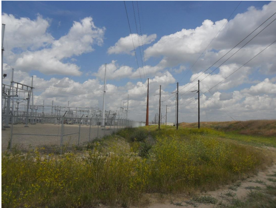
Photo 6 - Direction: North - Shows weeds along east fence
