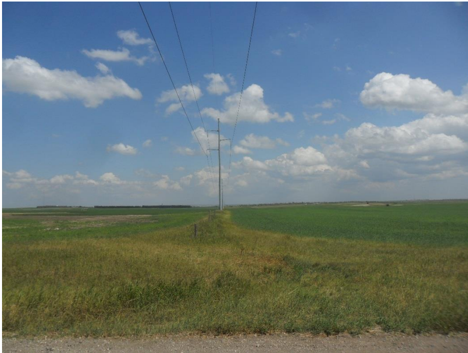
Photo 12 – Direction: East – Showing structures in section line to reduce crop loss
