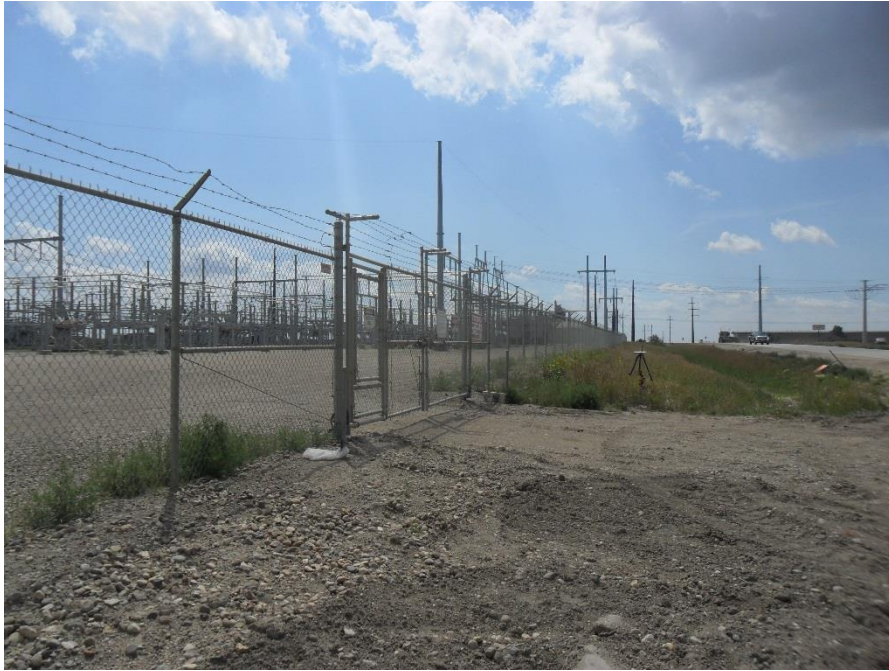
Photo 3 - Direction: South - Entrance to Williston Substation. Small clearance below gate could allow wildlife in.
