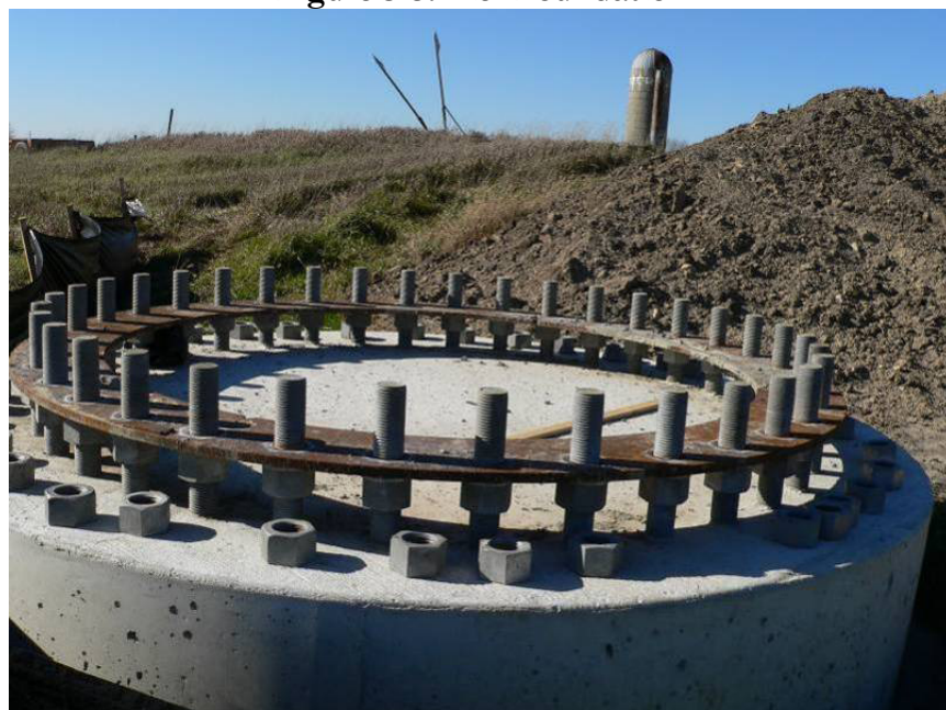
Figure 3-5. Pier Foundation
