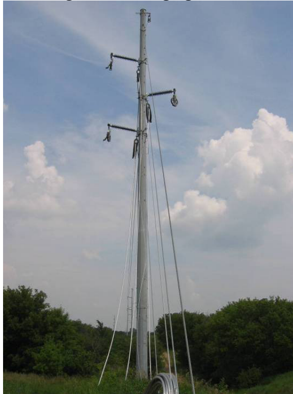
Figure 3-7. Stringing Process
