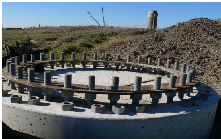
Figure 3-5. Pier Foundation
