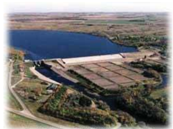
Aerial photo of Baldhill Dam and Lake Ashtabula, looking north.
