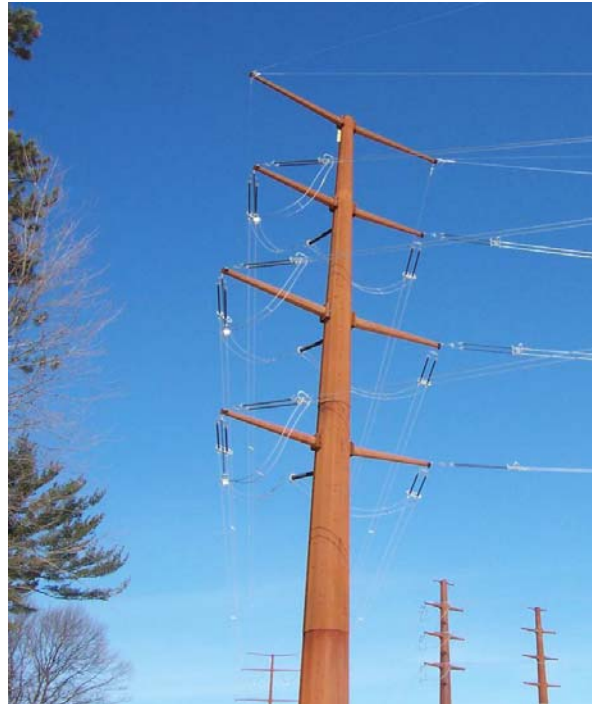
Figure 3-1. Representative 345 kV Double-Circuit Single Pole Structure (Self-Weathering)
