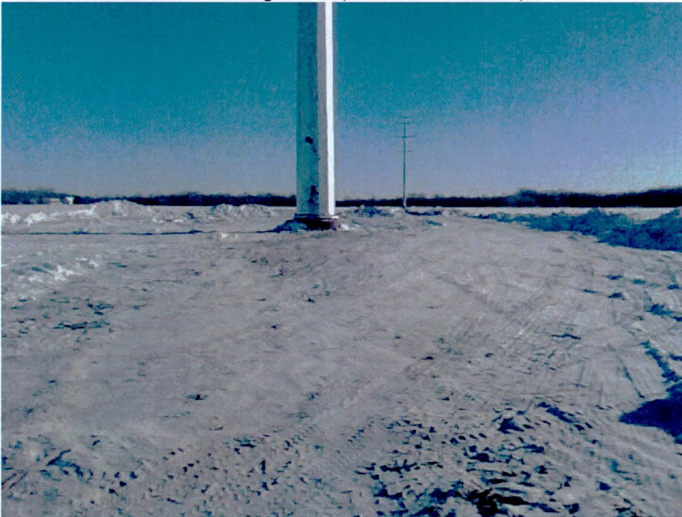
1/2/2014 – Structure #185 construction area. Ground is very frozen.
