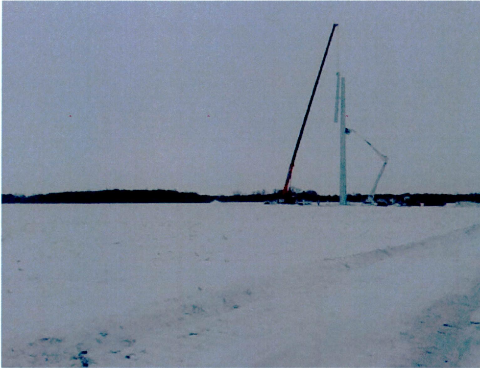
12/30/2013 – Structure #185 being erected (first tower on ND side)
