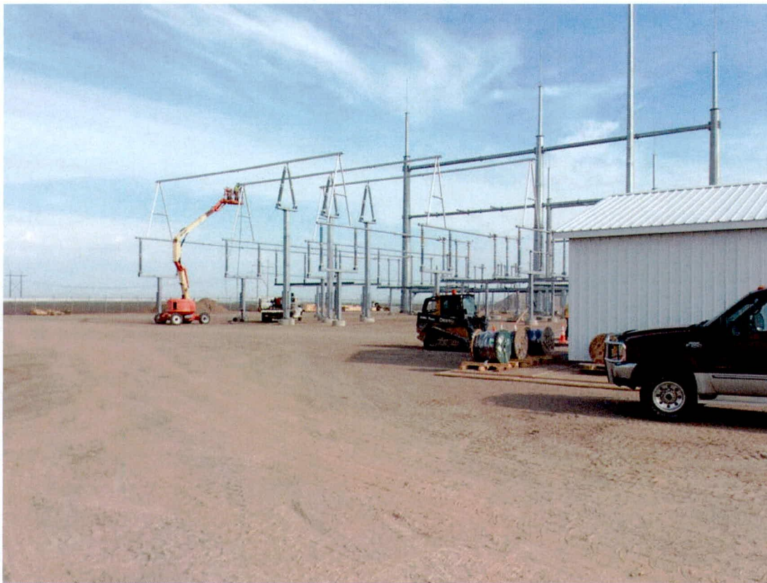
5/30/14 – Bison substation progress
