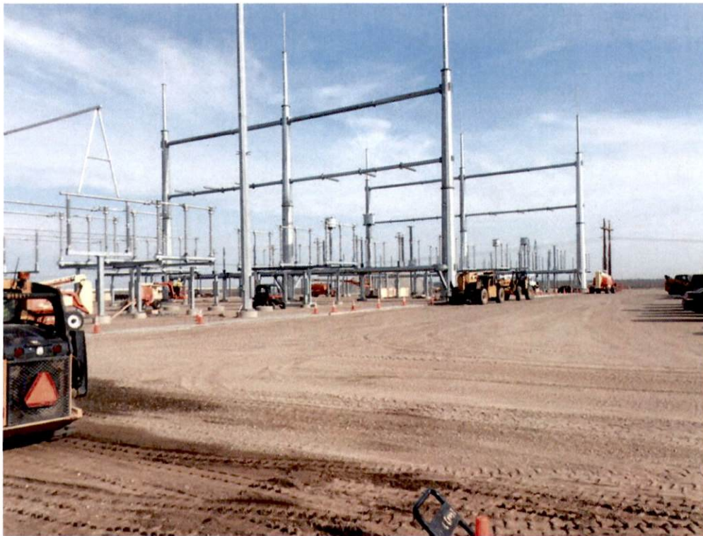
5/30/14 – Bison substation progress
