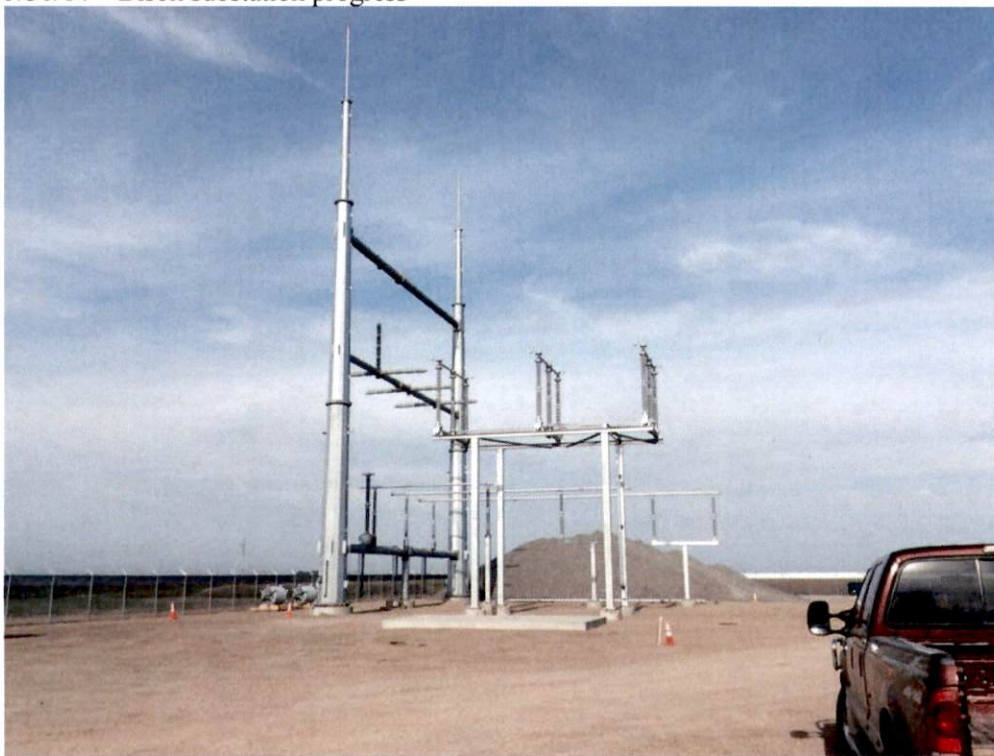
5/30/14 – Bison substation progress
