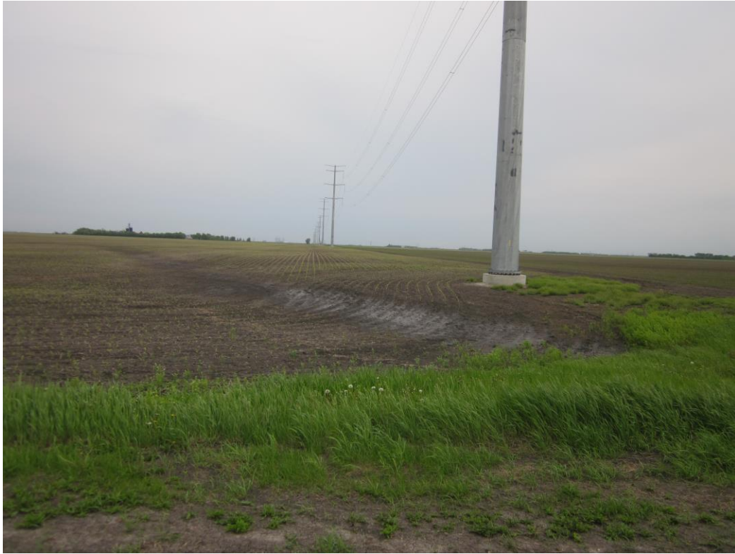
Above: Photo 5 – Transmission line through farm field.
