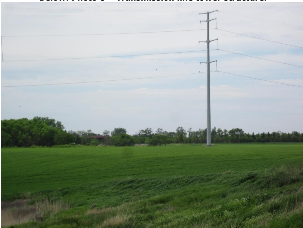
Below: Photo 8 – Transmission line tower structure.
