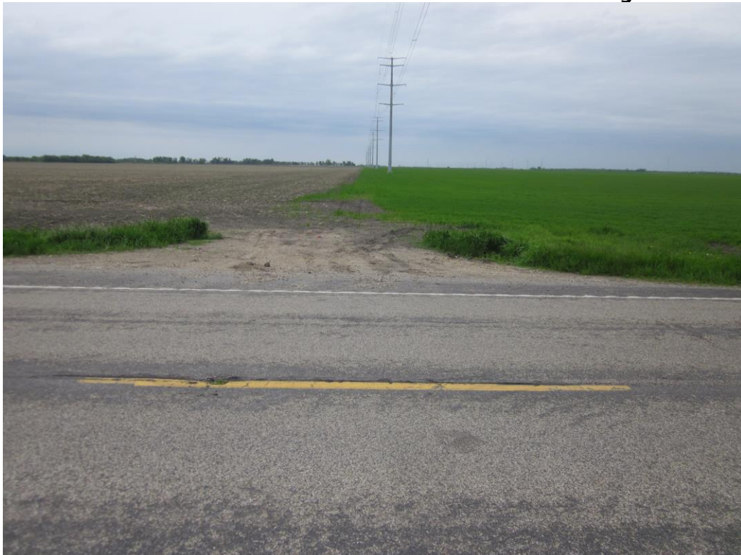
Below: Photo 6 – Transmission line road crossing.
