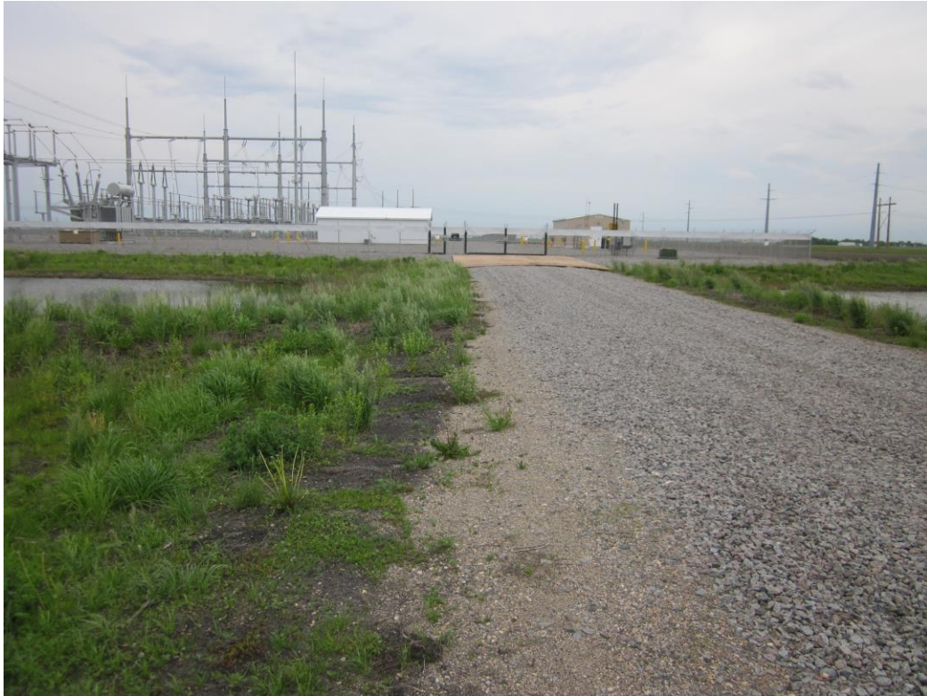
Above: Photo 1 – Bison switching station access road.
