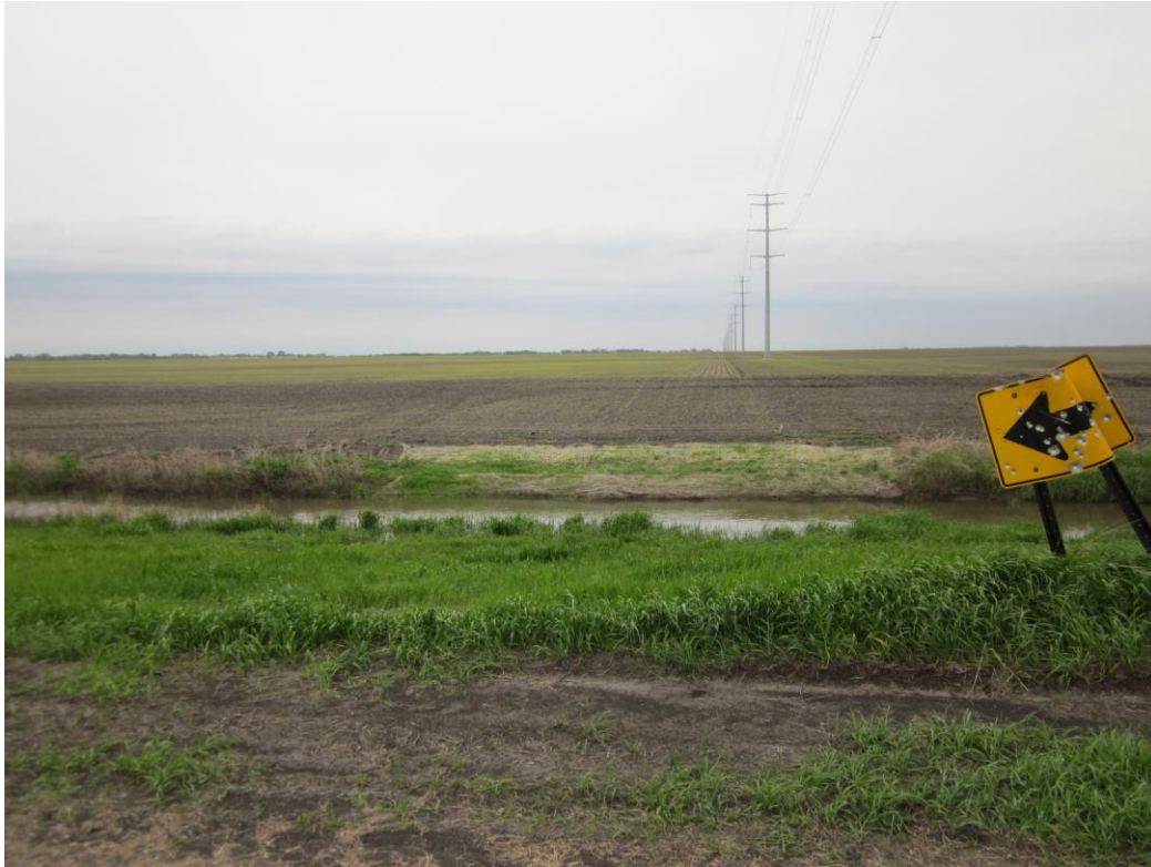
Above: Photo 7 – Transmission line through farm field.
