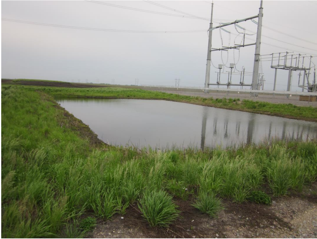
Above: Photo 3 – Transmission line leaving bison station.
