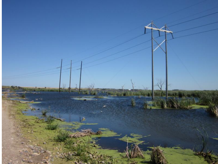
Photo 1. Direction: East/Southeast. West end of transmission line reroute. The H-frame structure in the right foreground was likely part of the original route. The three monopole structures on the left were the beginning of the reroute. The monopoles had guy wires attached. All structures were in standing water at the time of the survey.
