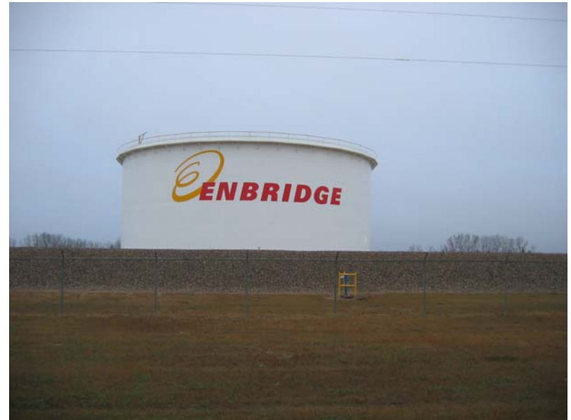
Minot Station. View of southern edge of facility and existing storage tank.
