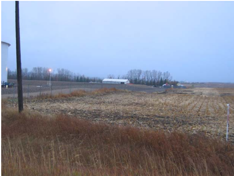
Minot Station. View along the northern edge of the facility.
