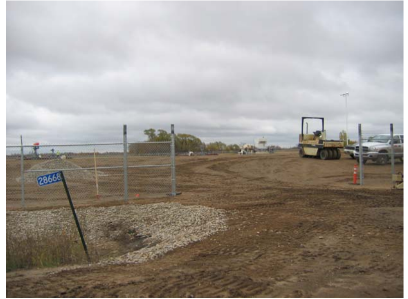
Brooks Station. Current activities at the station.
