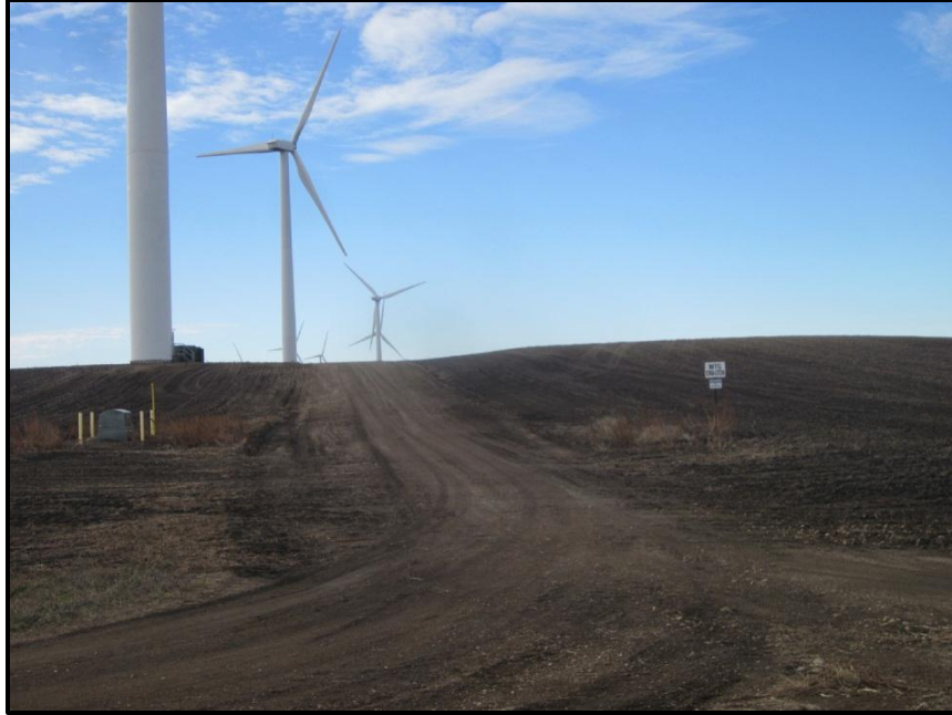
Photo 17. Direction: West. Access road for Otter Tail (OT) owned Turbines 48-39, at the intersection with 121 st Ave SE. The east half of the turbine string went through cropland and the west half went through rolling native prairie. Proper signs were in place. Roads, towers, junction box, and cropland were for the most part in good condition.
