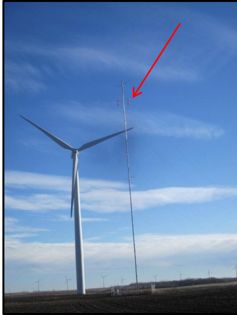
Photo 27. Direction: Southeast. MET tower to the northwest of Turbine 4. This tower had guy wires, but it also had the large orange balls on the wires as a bird deterrent (red arrow).
