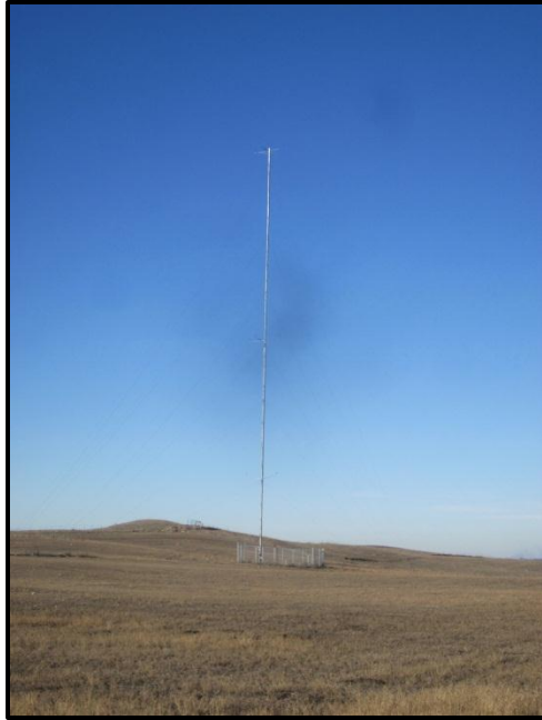
Photo 25. Direction: Northwest. MET tower to the northwest of Turbine OT34 in the NW ¼ of Section 6, T142N, R57W. The tower had guy wires. No known birdsafe design features were visible.
