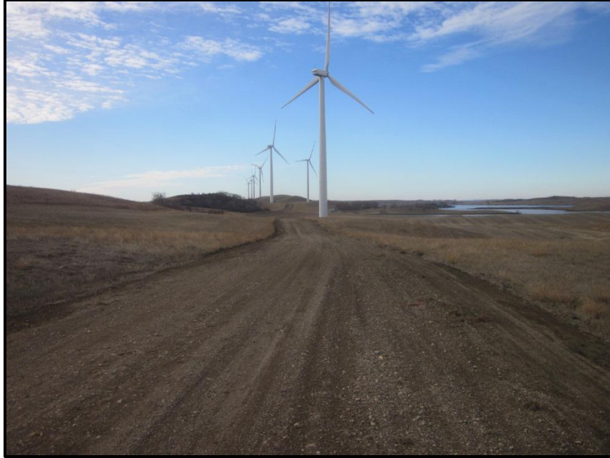
Photo 19. Direction: West. Road near Turbine OT46 showing the rest of the string across rolling hills. The road edges did not appear to have been planted with grass during reclamation. Rather the adjacent, existing hayland of alfalfa appeared intact up to the edge of the road; it appeared to have not been disturbed during construction or it had naturally grown back in since being disturbed.
