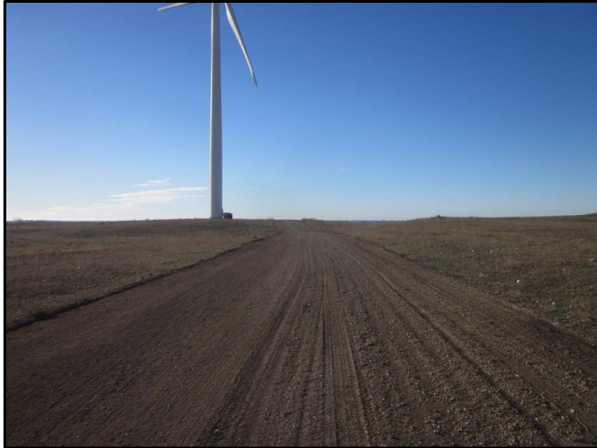
Photo 23. Direction: West. Access road leading to Turbine OT39. Conditions were good with no concerns. The native prairie along this portion of the access road did not appear to have been disturbed during construction; however there did appear to be drill rows in the soil and vegetation.
