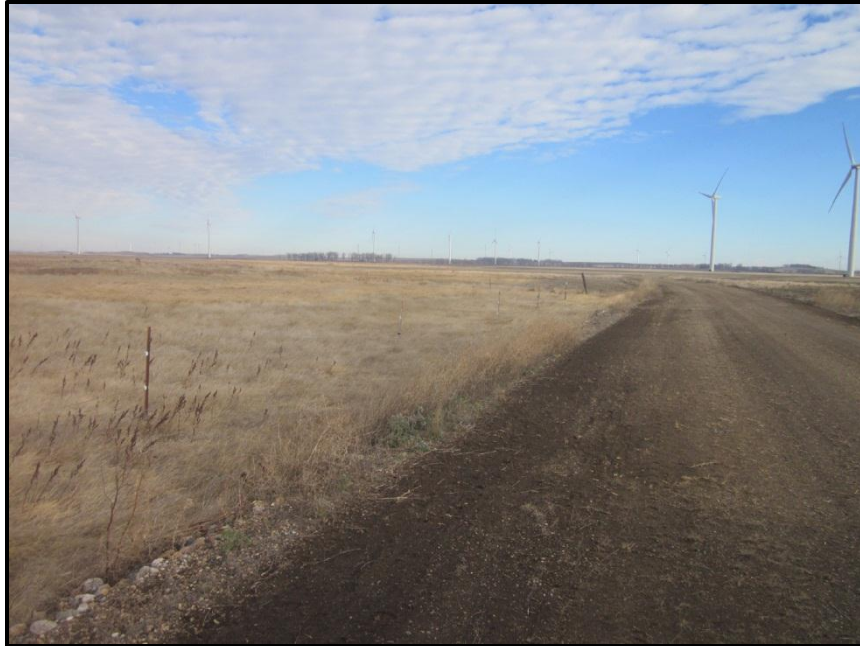
Photo 13. Direction: North. Access road along Turbine string 105-108, which was sited to avoid a low prairie/wetland complex to the north and west. It did not appear that the edges of the road had been disturbed beyond the actual road width during construction and thus had not been reseeded.
