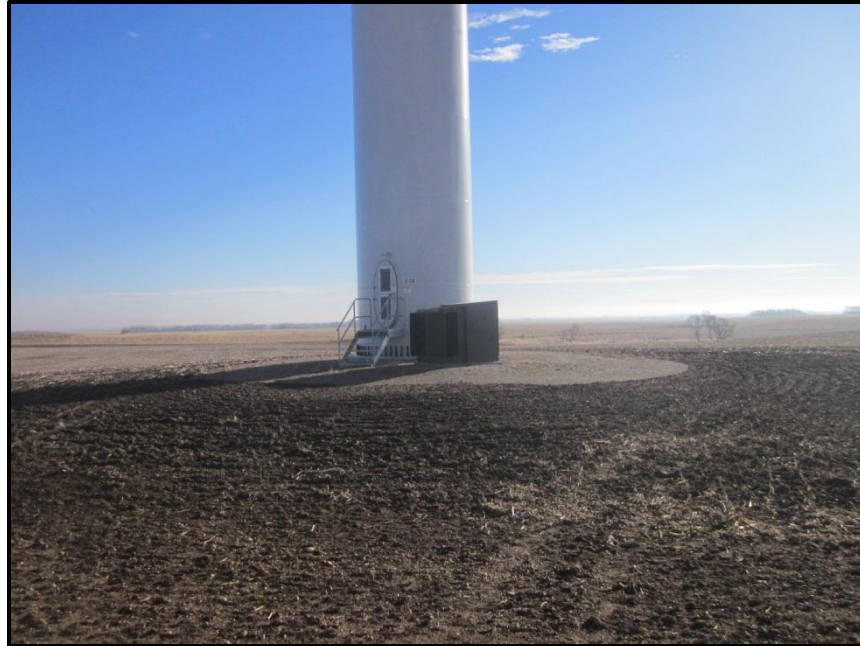
Photo 11. Direction: Southeast. Base of Turbine 126. The landowner had tilled through the gravel pad here and at Turbines 125 and 127, ruining the gravel surface and preventing access to the tower. NextEra was actively addressing the issue, since landowners have agreed not to disturb the gravel maintenance pad as part of the lease agreement with the wind company.
