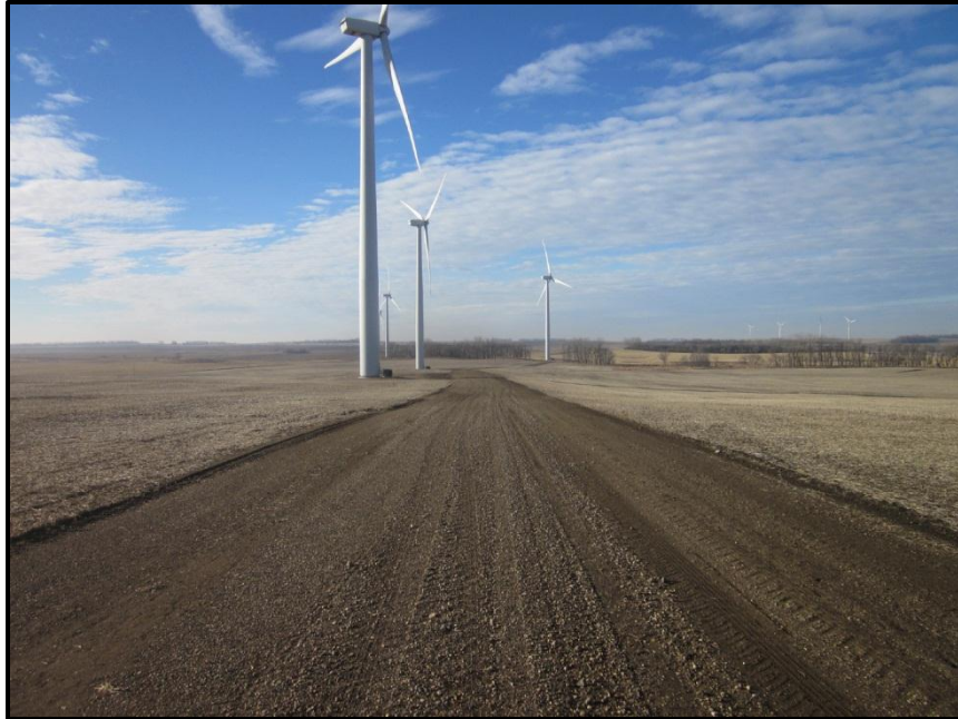
Photo 7. Direction: Southwest. Continuation of access road along turbine string 131-125. Turbines, roads, and cropland were all in good condition with no concerns.
