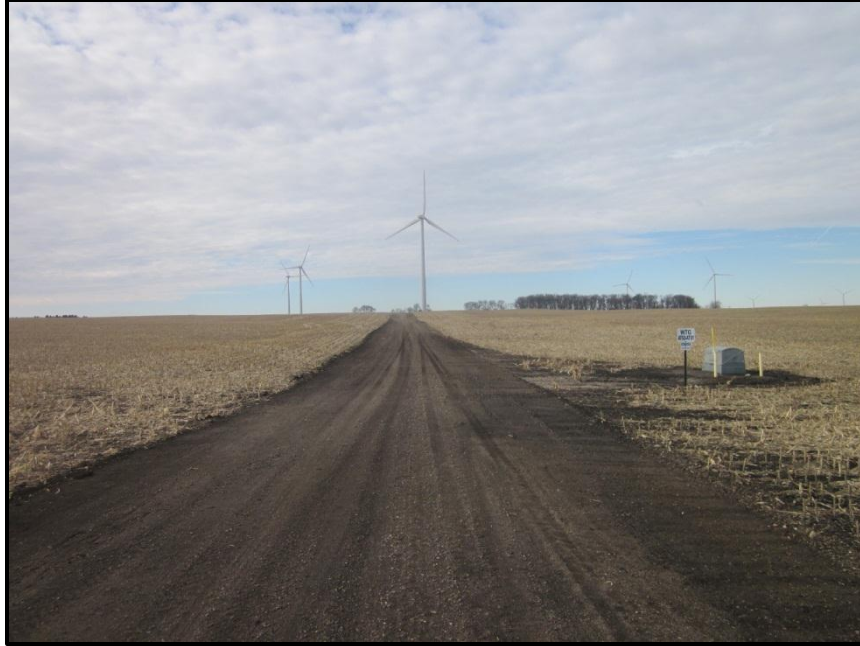
Photo 15. Direction: West. Access road entrance to Turbines 93-91 through cropland. Proper signs were in place. Cropland, roads, junction box, and towers were in good condition. This turbine string was on land under USFWS wetland easement. All drainages and wetlands had been avoided.
