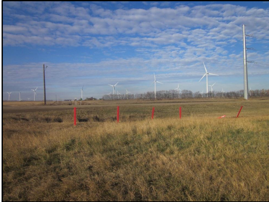
Photo 5. Direction: West. Series of red markers noting locations of numerous underground collection lines leaving the substation from its southwest corner. The lines had been bored underneath County Road 27, visible beyond the ditch running north-south. Several turbine strings for Ashtabula I are visible in the distance.
