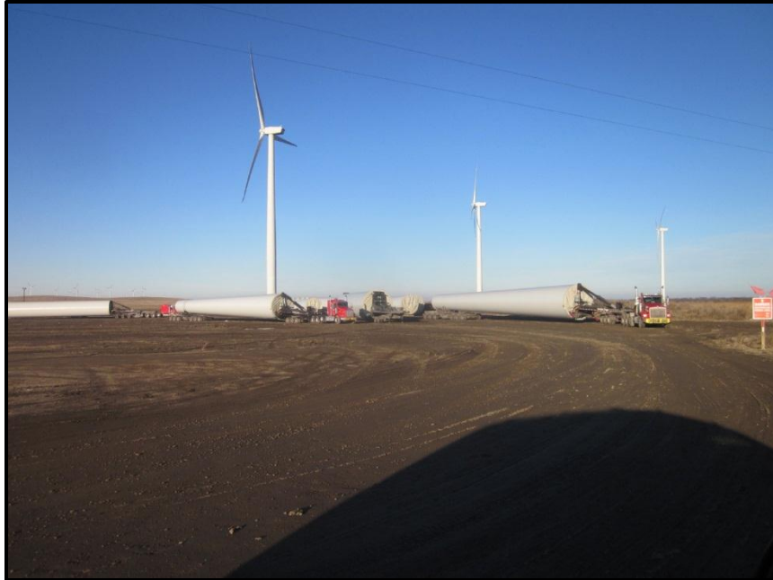
Photo 3. Direction: Northeast. Far eastern side of laydown area where tower sections were being moved by semi-truck at the time of the site visit. Note the safety sign on the far right of the photo warning of overhead power lines. Turbines 63-65 are visible in the distance.
