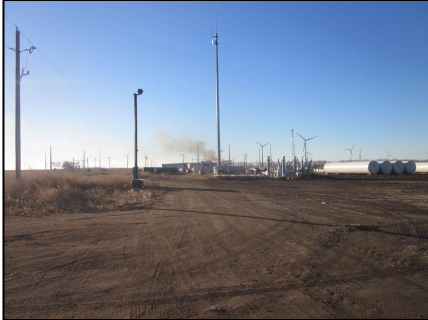
Photo 1. Direction: West. View across the O&M building and laydown grounds from the east side to west side, located in the southwest corner of Section 10, T142N, R57W. The east side of the grounds in the foreground, along with the north side (not visible), was still being utilized for construction and staging purposes. Maintenance and operations activities and equipment were situated around the O&M building in the distance on the west side of the grounds.
