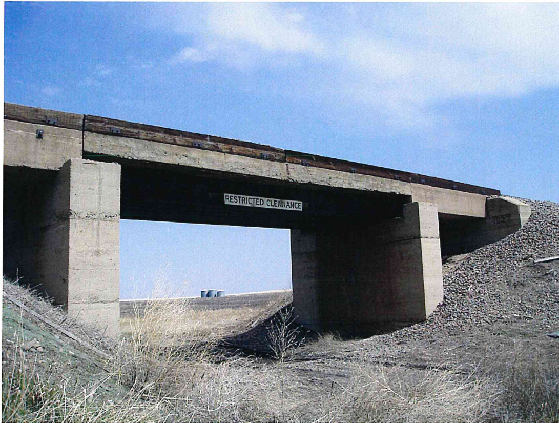
Figure 2: The railroad bridge. Photo taken looking northeast.
