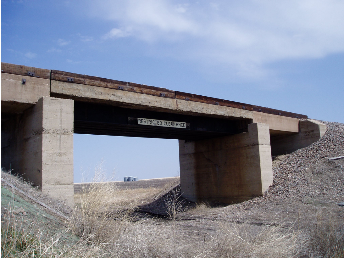
Figure 2: The railroad bridge. Photo taken looking northeast.
