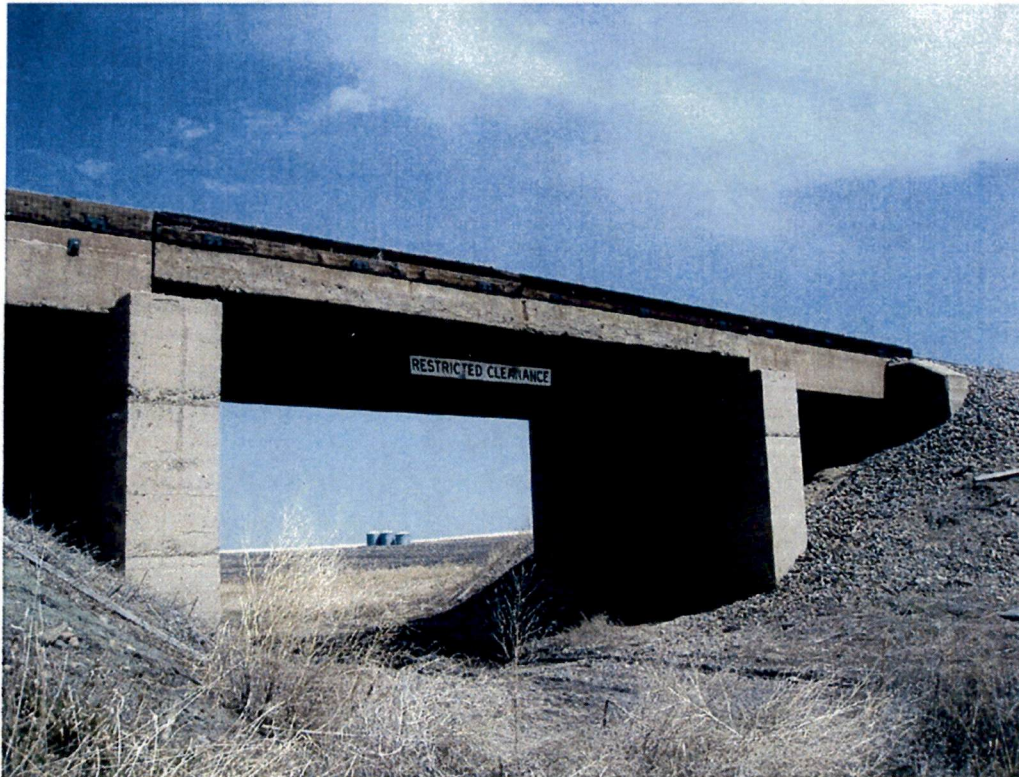
Figure 2: The railroad bridge. Photo taken looking northeast.
