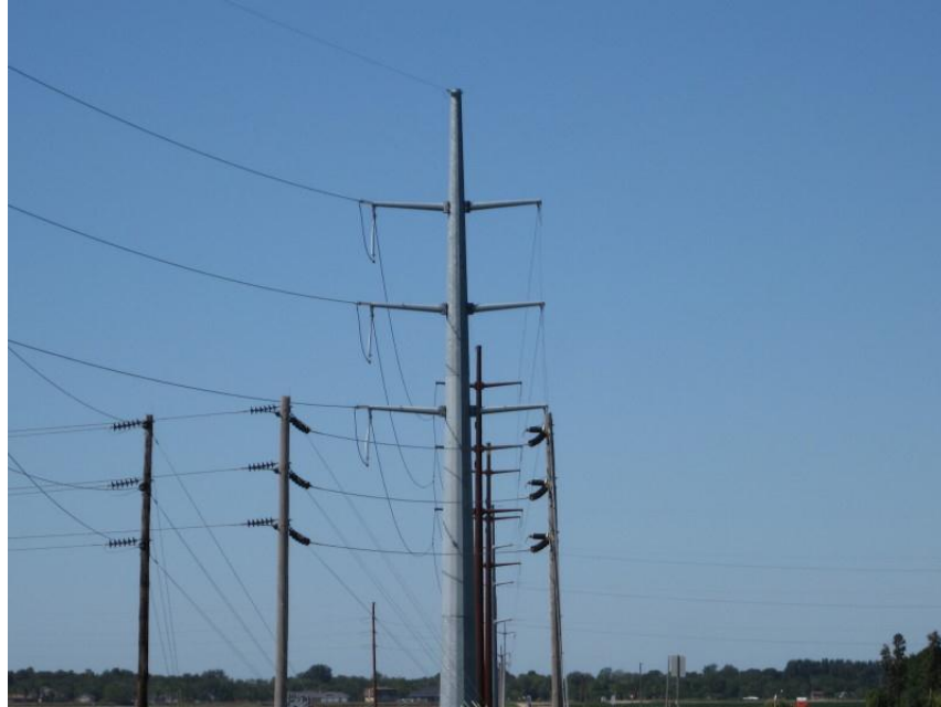
Photo 29. Direction: West. Monopole at end of transmission line as it entered the Maple River substation. The last portion of the line paralleled the south side of 32 nd Ave to the west of the substation.
