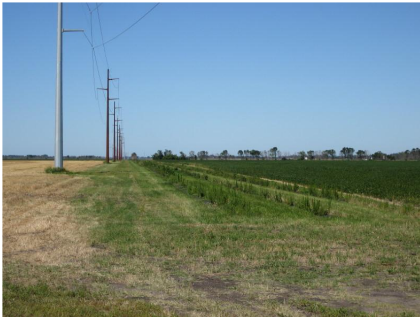
Photo 18. Direction: West. Intersection of transmission line with 153 rd Ave. Note planted tree/shrub rows on right which was one of the replacement plantings for the Project. This was located through the center of Section 33, T142N, R52W and appeared to be in good condition.
