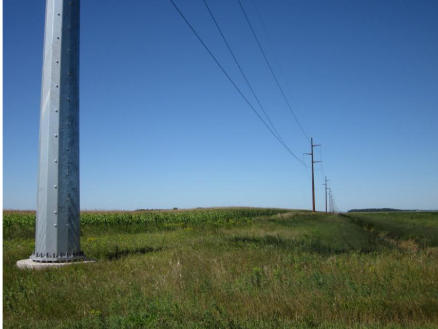
Photo 19. Direction: West. Transmission line where it paralleled 24 th St for several miles. 24 th St was a sectionline which had portions with no roads and portions with minimum maintenance two-track roads. This portion of the route primarily spanned active cropland.
