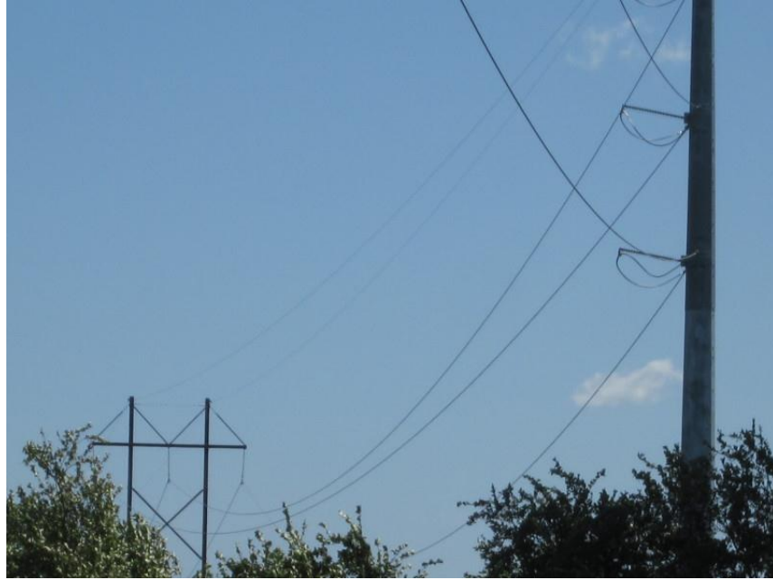
Photo 27. Direction: East. To the east of the crossing of the Sheyenne River, the 230 kV line runs back on a monopole structure (on right of photo), then to two H-frame structures (on left of photo), then back to monopoles. Note the trees in the photo appear to be close to the wires but this was due to the angle of the photo; they were not in need of clearing away from the line.
