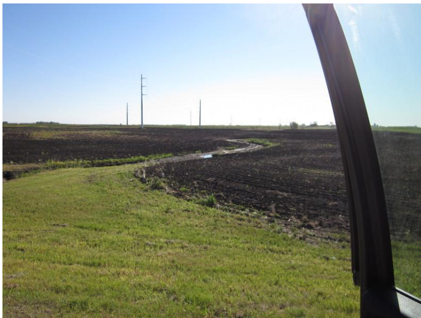
Photo 4. Direction: East. Intermittent drainage exiting underneath the approach for the Pillsbury substation entrance. According to Minnkota, the approach had been washed out and had to be reconstructed this past spring. There were no erosion control structures evident.
