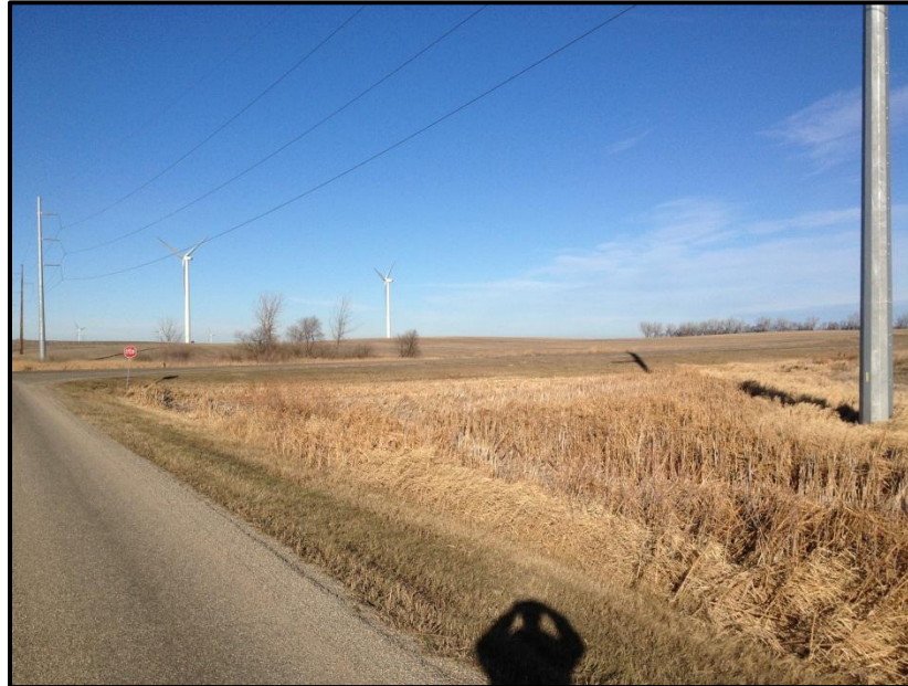
Photo 8. Direction: Northeast. At the intersection of ND Highway 26 and 123 rd Ave. SE, two wetlands were spanned in the ditches north and south of the Highway. Poles were in upland with no impacts to the wetland area.
