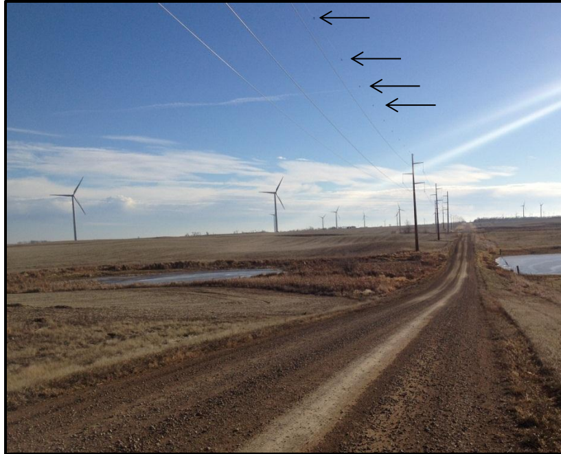
Photo 7. Direction: Southeast. View of wetland crossing along the transmission line route. It appeared the transmission line poles were in upland, with no apparent impacts to the wetland area. There were flight diverters along this portion of the route (indicated by black arrows).
