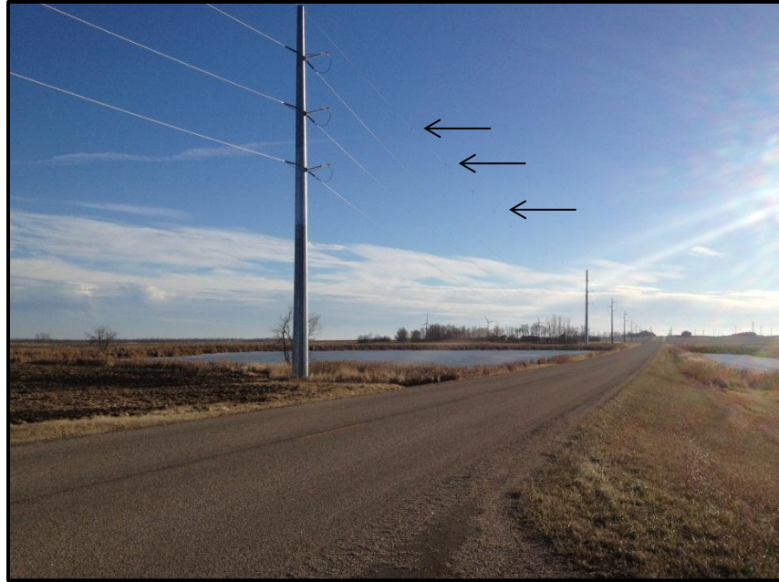
Photo 9. Direction: Southeast. View north of a water body crossing in Section 34, Township 143 North, Range 57 West. Structures were in upland with no impacts to the wetland area. There were flight diverters along this portion of the route (indicated by black arrows, but faintly visible).
