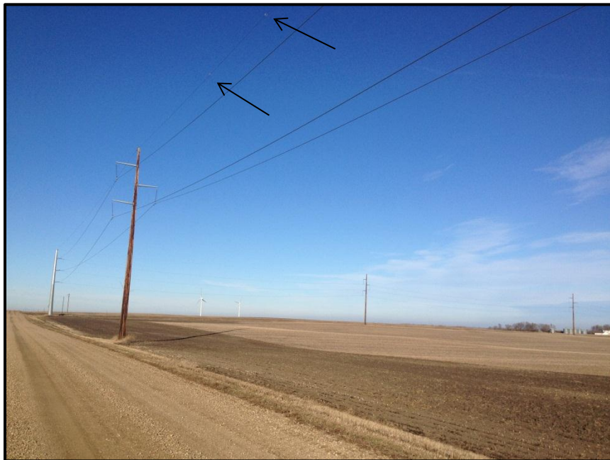
Photo 6. Direction: Northwest. View shows the transmission line as it turned north/south down 123 rd Ave. SE. There were flight diverters along this portion of the route (indicated by black arrows).
