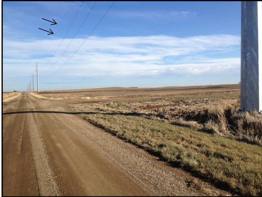
Photo 3. Direction: East/Southeast. View shows the transmission crossing nearby Goose Lake. The landowner appeared to have mowed the wetland vegetation prior to the inspection. The pole on the right of this photo is upland, with no apparent disturbance to wetland vegetation. There were flight diverters along this portion of the route (indicated by black arrows, but faintly visible).
