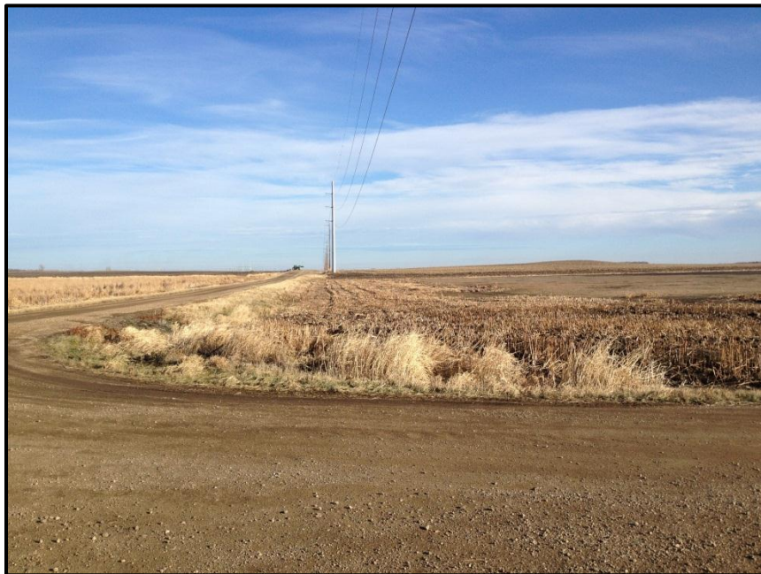
Photo 4. Direction: East. Another view of the transmission line spanning the wetland area south of Goose Lake.
