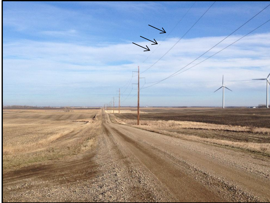
Photo 5. Direction: East. View of the transmission line as it went east-west down 14 th St. SE. There were flight diverters along this portion of the route (indicated by black arrows).
