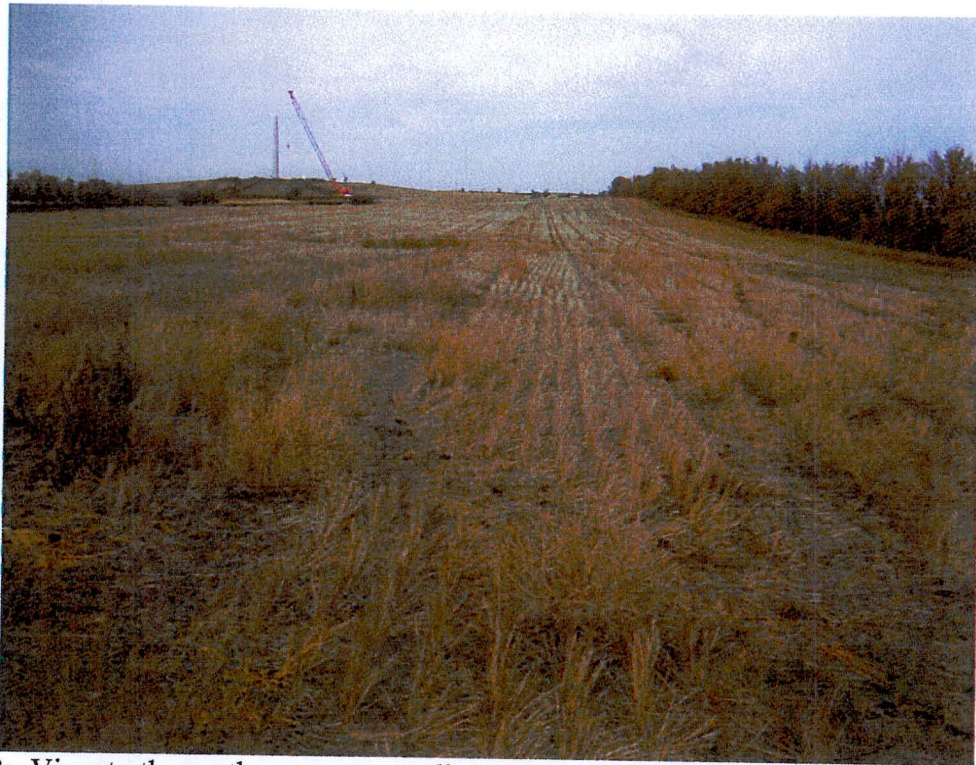
Figure 2: View to the north over crane walk, note crane in background (Image 10-26-09, 19).
