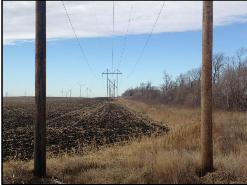
Photo 9. Direction: West. The tree row to the right had been cut to accommodate the transmission line and it appeared impacts to the area had been minimized. Note the flight diverters that were installed in this area.
