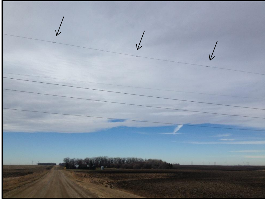
Photo 7. Direction: Northwest. View shows typical bird diverters installed at several areas along the transmission line (indicated by black arrow).
