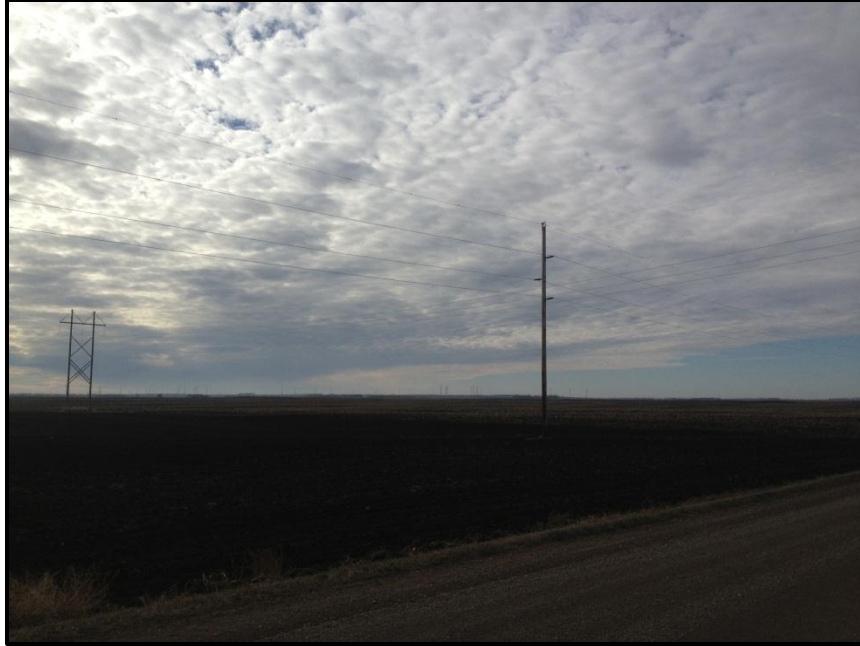
Photo 5. Direction: Southwest. View of the transmission line (H-frame structure on left) crossing Minnkota's Keystone line (single pole structure).
