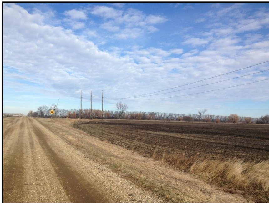
Photo 2. Direction: North/Northeast. View shows the transmission line just north of the substation as it runs parallel to 126 th Ave SE in Barnes County, ND.
