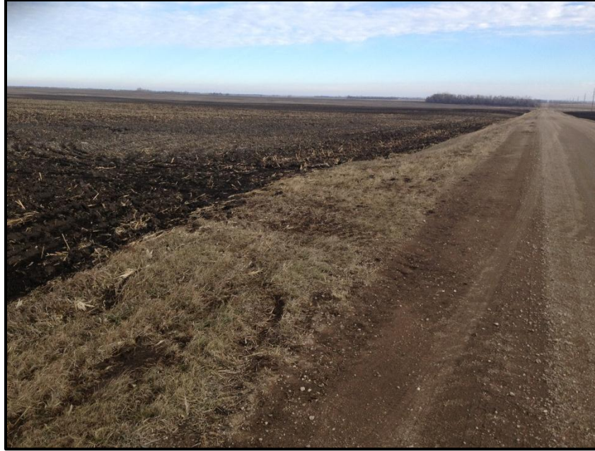
Photo 11. Direction: Northeast. View of a typical reclaimed access road used for the Project. Vegetation had established along the road ditch. No disturbance was noted in the agricultural field.
