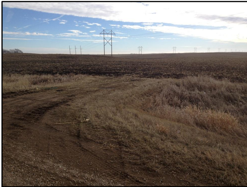
Photo 12. Direction: Southeast. This access road had been retained by the landowner for access to the agricultural field. No disturbance from access road construction was noted in the agricultural field.
