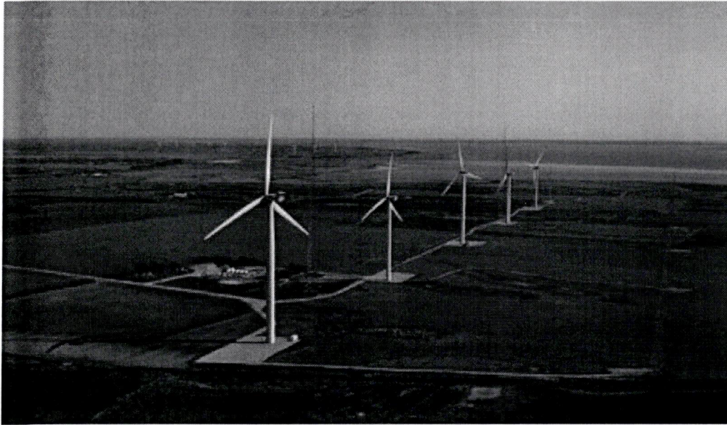
Figure 1: Aerial view from north of Høvsøre Test Site. The SWT-2.3-93 is fifth in the row (right)
