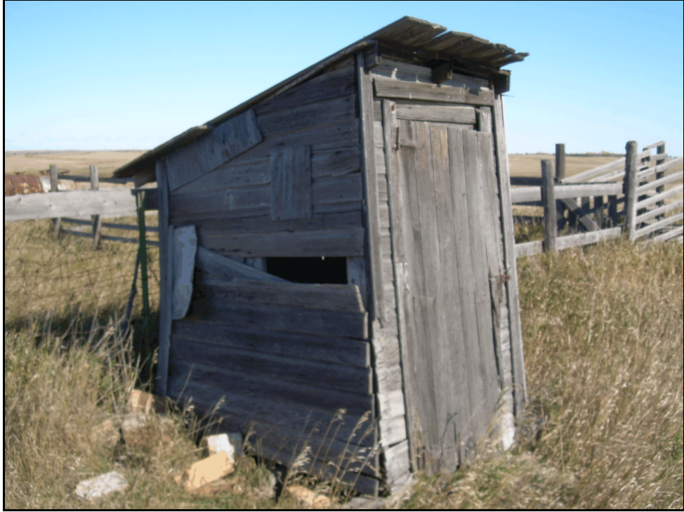
Figure 25 View to the northeast over Features 1 and 2, 32MN775 (image 479).
