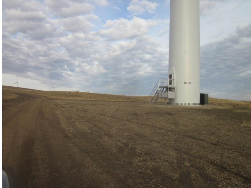
Photo 3. Direction: Northwest. Typical turbine pad and turbine for the project; Structure 1-30 is shown here. The gravel pad was well maintained and free of noxious weeds.
