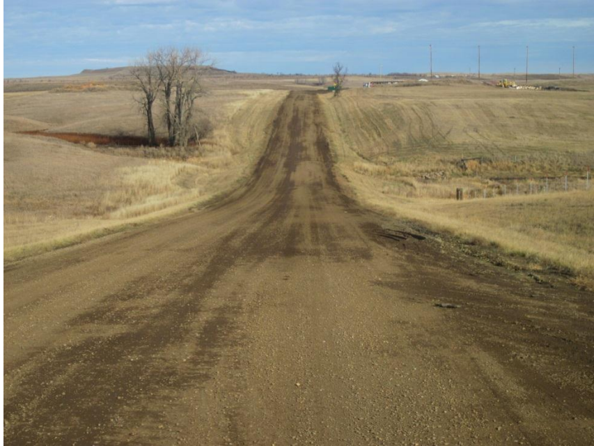
Photo 11. Direction: North. View of 52 nd Ave, which had been improved by Minnesota Power and was currently in good condition and well maintained. This was typical for roads in the project area. Reclamation of the road margins was successful, as evidenced by establishment of vegetation.
