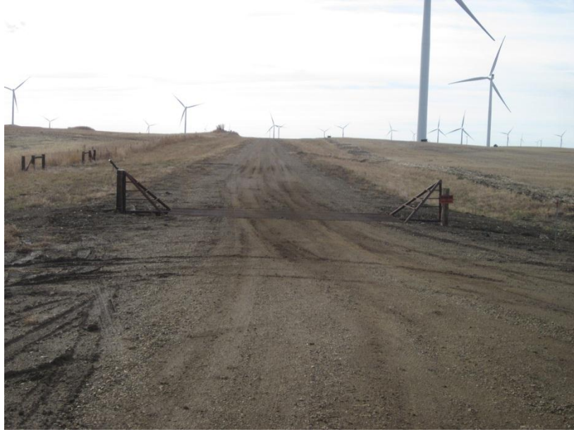
Photo 9. Direction: South. Cattle guard installed along access road.
