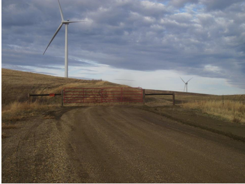
Photo 1. Direction: West. Access road and cattle guard for Structures 30, 2, 10, 1, and 27; Structures 30 (left) and 2 (right) are shown here. The access road was well maintained, and road margins appeared to have been reclaimed with native species successfully.
