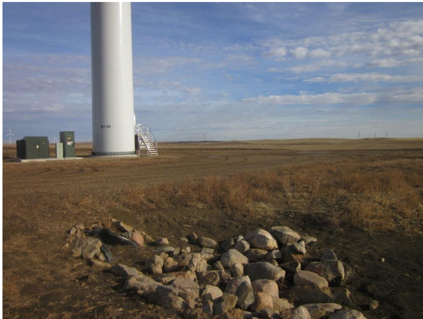
Photo 12. Direction: South. Structure 29 with associated culvert.
