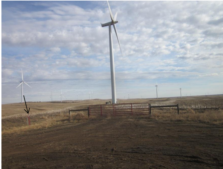
Photo 10. Direction: Structure 32 with associated access road, gate, and feeder line marker (black arrow).
