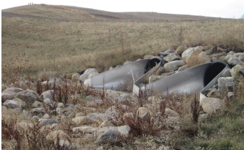
Photo 6. Direction: Southwest. Culverts installed along access road to Structure 26.
