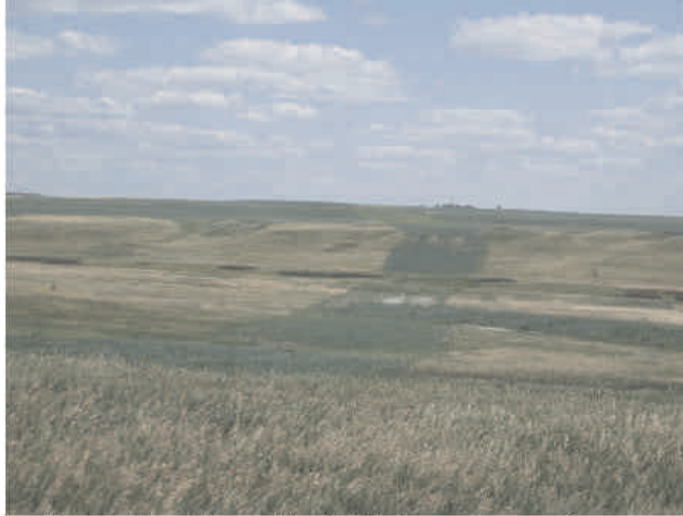
Figure 5: Looking east from the west bank. The large green swatch represents previous pipeline construction.
