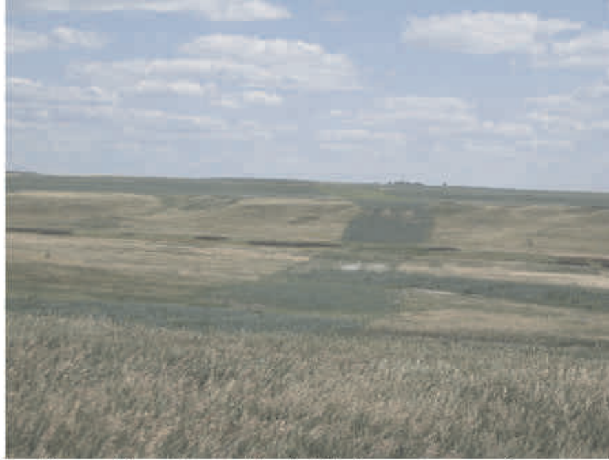
Figure 5: Looking east from the west bank. The large green swath represents previous pipeline construction.
