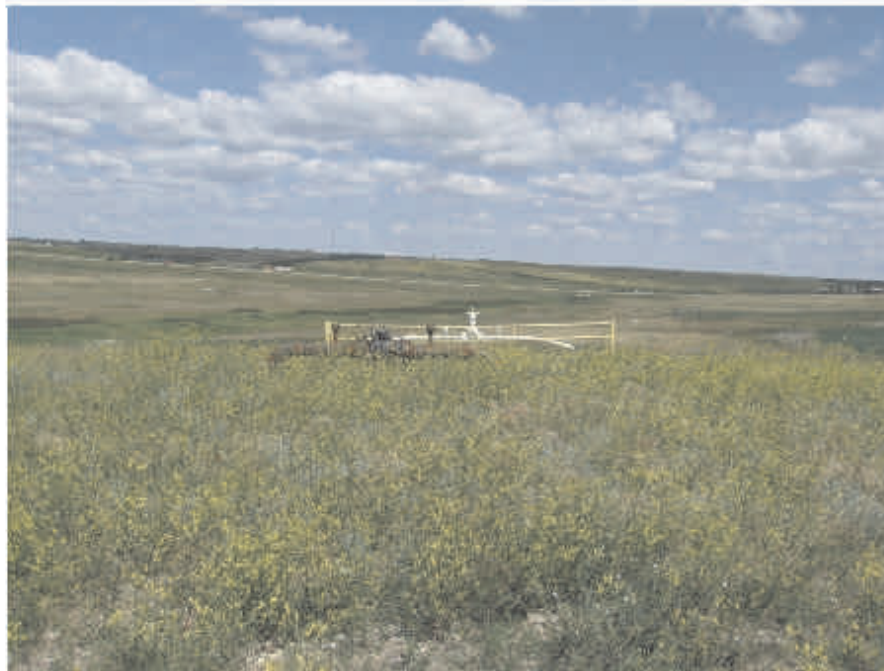
Figure 3: Looking to the northwest from the top of the east bank. The Embridge Pipeline is in white and the second unmarked pipeline is in brown.
