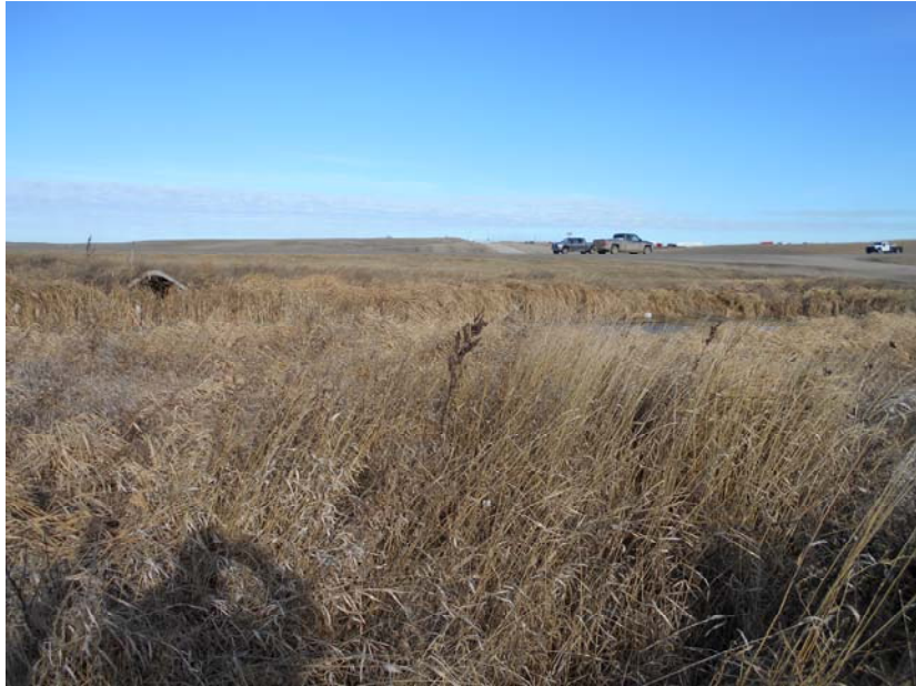
Photo 17 – Direction: North –Pipeline crossing Highway 2, Stanley, ND. No pipe marker was able to be located in this area marking the pipeline crossing located just south of Highway 2, Stanley, ND
