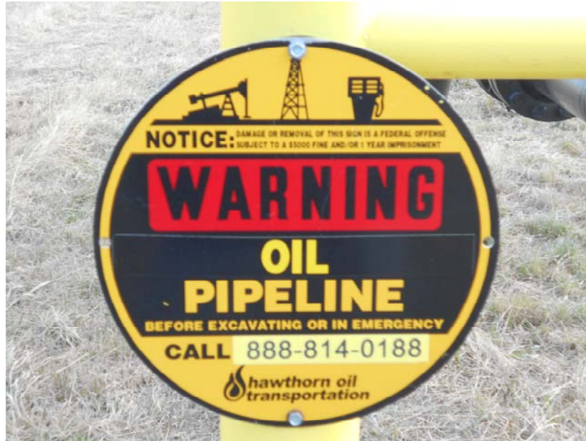
Photo 7 – Direction: East – Pipeline marker on west valve station before crossing Little Knife River.
