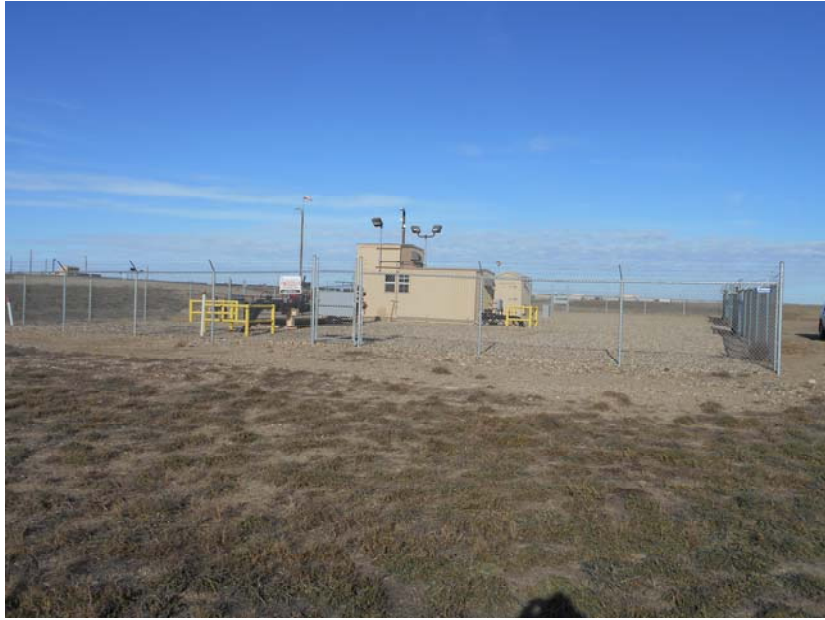
Photo 23 – Direction: North – Valve Station north of Highway 2, Stanley, ND.
