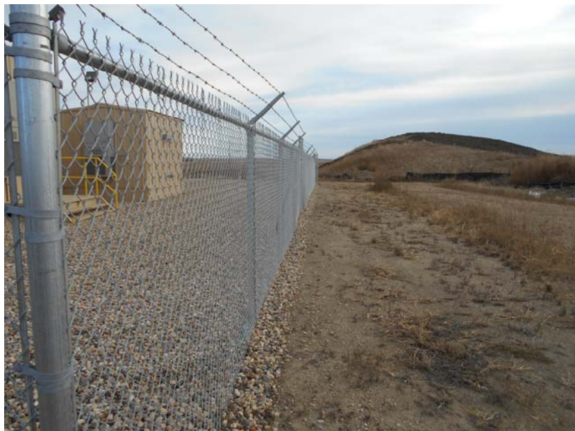
Photo 4 – Direction: East – Showing perimeter fencing on valve station.
