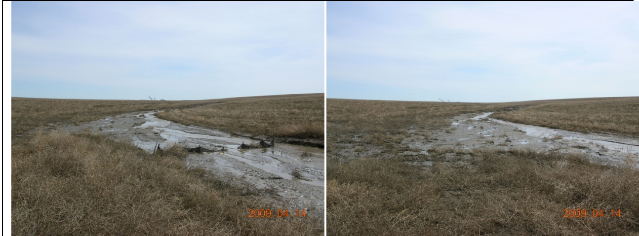
Drainageway in SW¼ of Section 13, Permit KRSB-8802. Sediment deposition on reclaimed lands.
