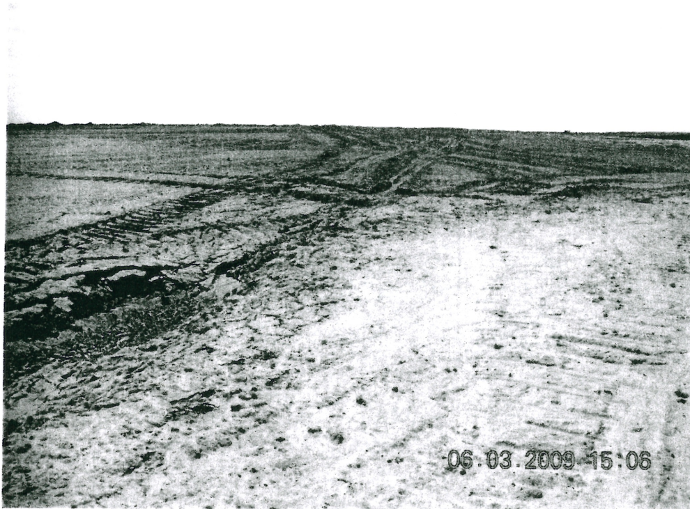
Looking west at ruts and differential settling along the north edge of GA W28A.
