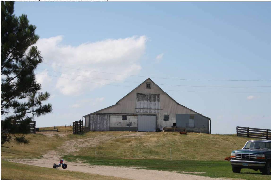
Photograph 33. TTAW 14 -- T131N, R69W, Sec. 21. Photograph looking west. (James Sexton, Tetra Tech, July 17, 2010)
