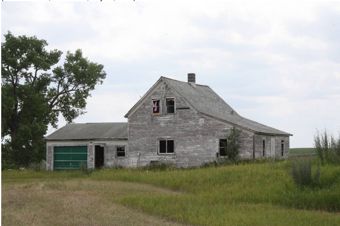
Photograph 8. TTAW 5 -- T131N, R70W, Sec. 12. Photograph looking west. (James Sexton, Tetra Tech, July 17, 2010)
