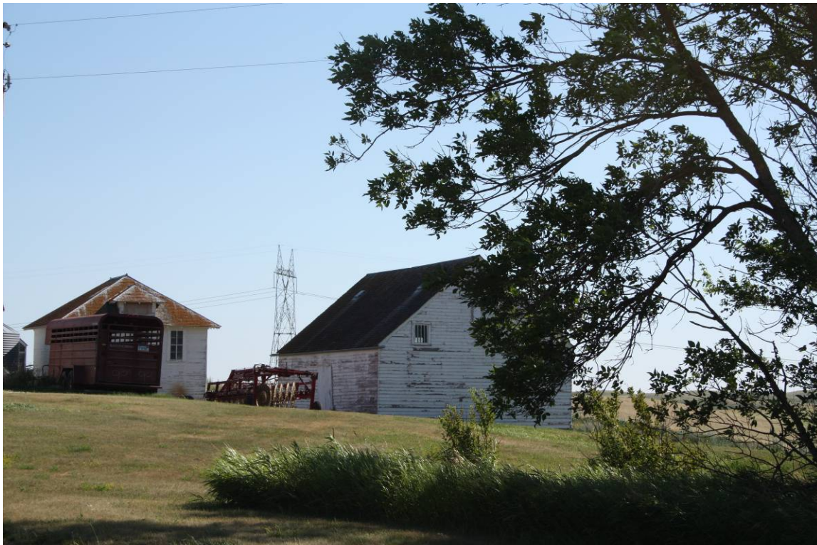
Photograph 26. TTAW 9 -- T131N, R69W, Sec. 11. Photograph looking southwest. (James Sexton, Tetra Tech, July 17, 2010)
