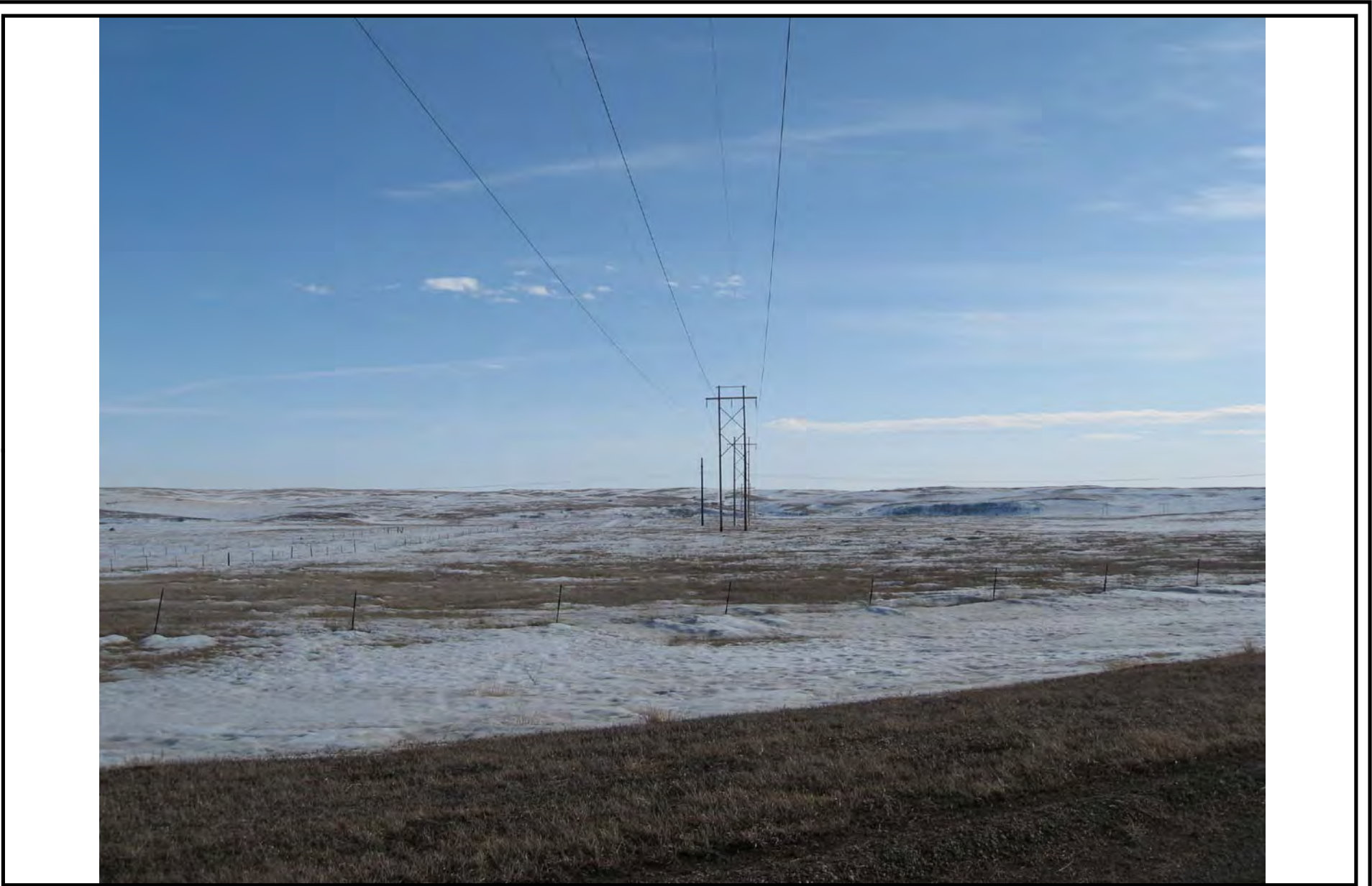
Figure 10: Existing Environment Proposed Transmission Route Bison I Wind Project, Minnesota Power Morton & Oliver Counties, ND
