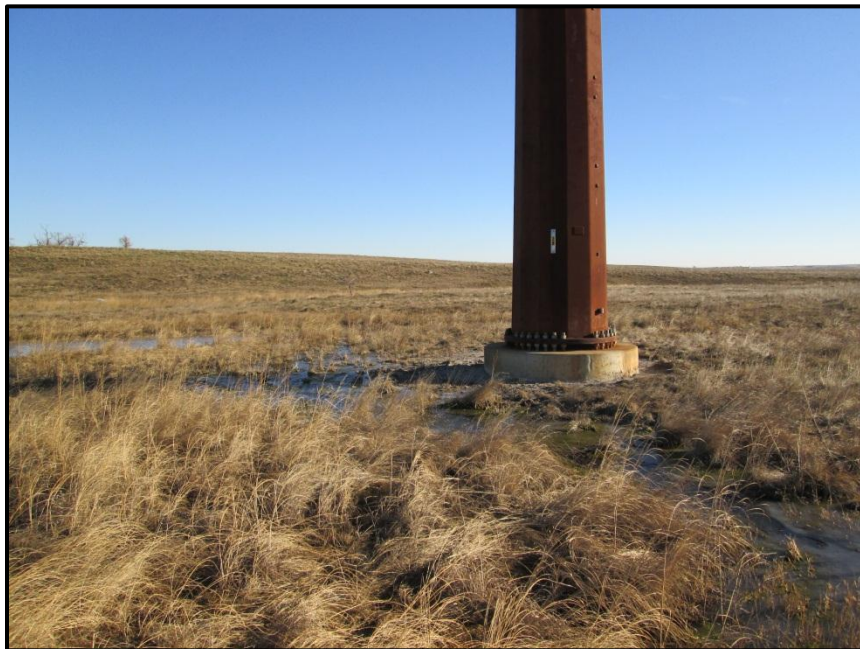
Photo 6. Direction: East. View of a transmission structure within a wetland. Disturbance to the wetland was minimized to the extent possible. Wetland vegetation had reestablished and no residual sedimentation from construction was observed. A mitigation wetland was created to mitigate wetland impacts (Photo 10).
