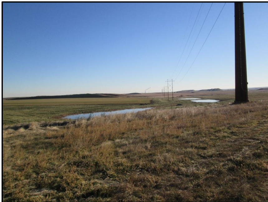
Photo 4. Direction: East. View of the transmission line as it spanned a wetland area west of the Center Mine. The transmission poles were in upland areas and no construction-related disturbance to the wetland was noted.
