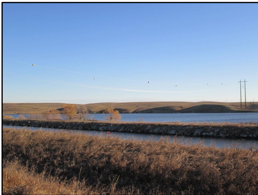
Photo 2. Direction: Northeast. View of the transmission line as it crossed Lake Nelson. Bird diverters were installed on the transmission line around the lake.
