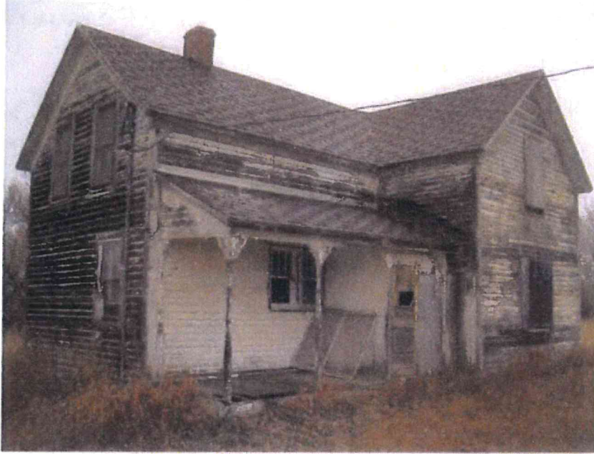
Figure 4: View southeast to northwest, Feature 1 at site 32BL655. (Image #15)
