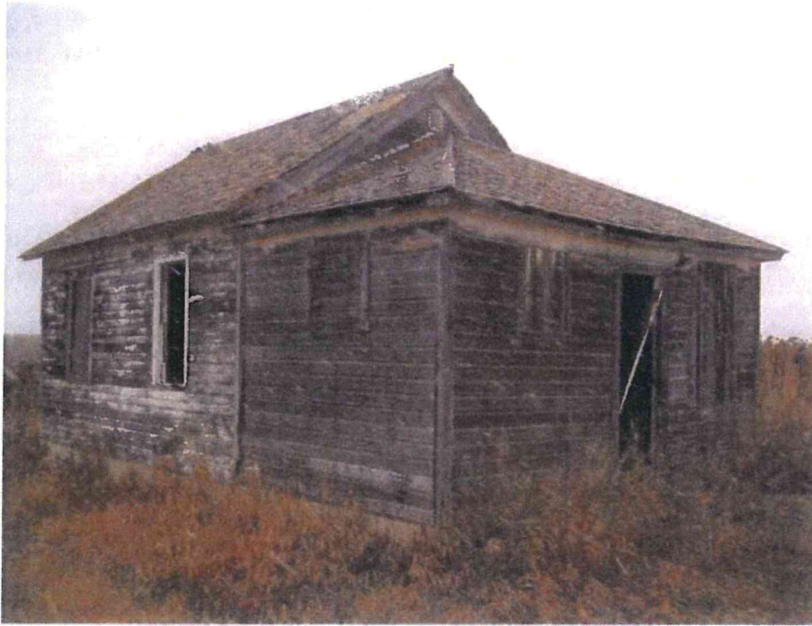
Figure 2: View southwest to northwest over site 32BL654 (Image #001)
