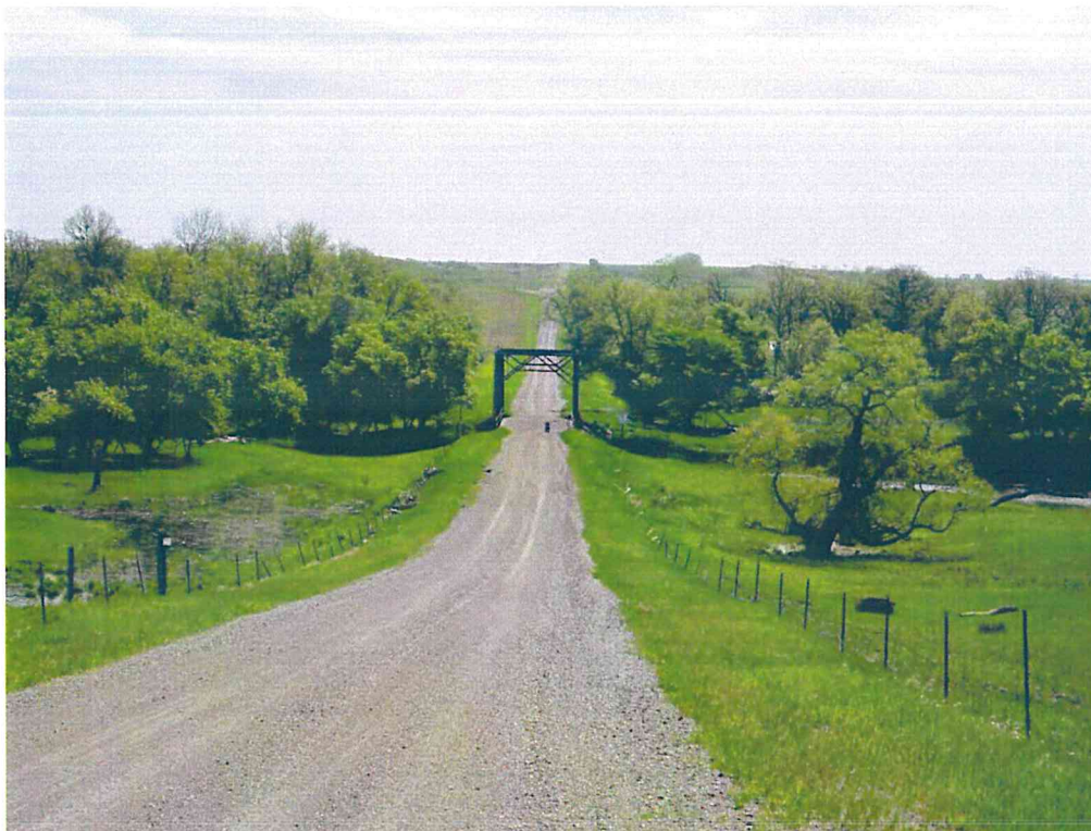
Photo 4 – Sheyenne River Crossing
