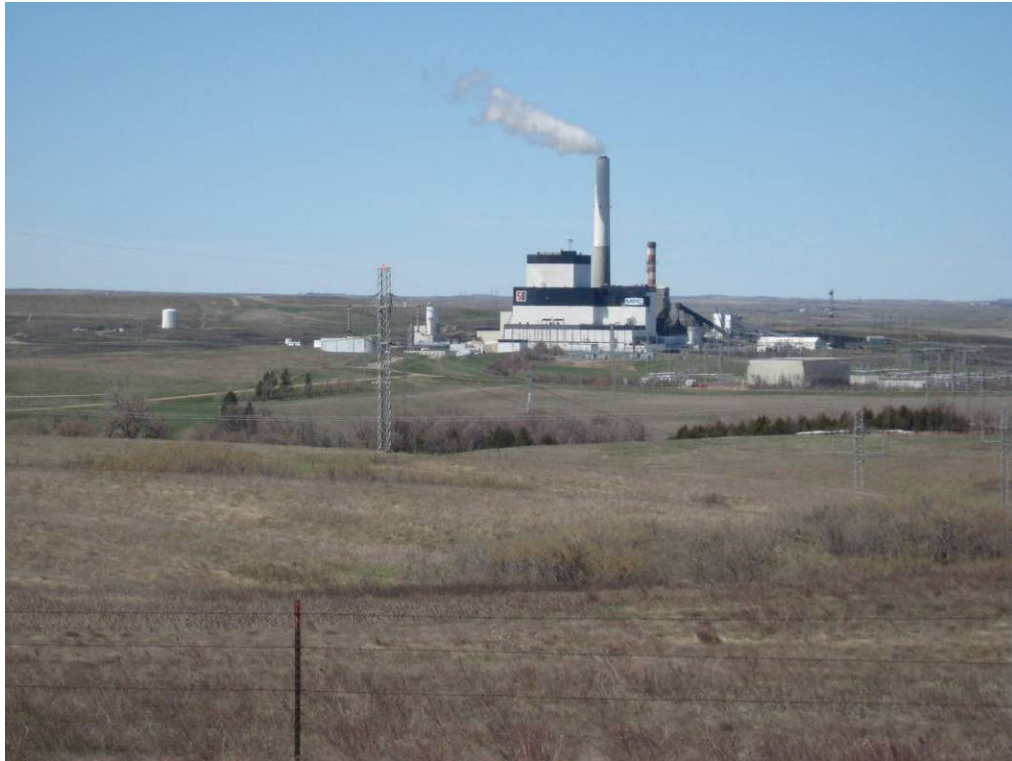
Photo 1 – Milton R. Young Station near Center, North Dakota
