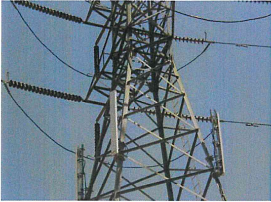
Cellular antennas and equipment sheds utilize transmission lines.
