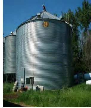
Modern vintage GSI company bin HDR 11932/41403 Rosefield Township, Eddy County
