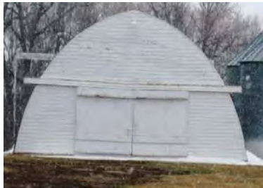
Wood style Quonset building site lead 39998 Wells County
