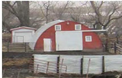
Wood style Quonset building site lead 17606/41874 Sheridan County
