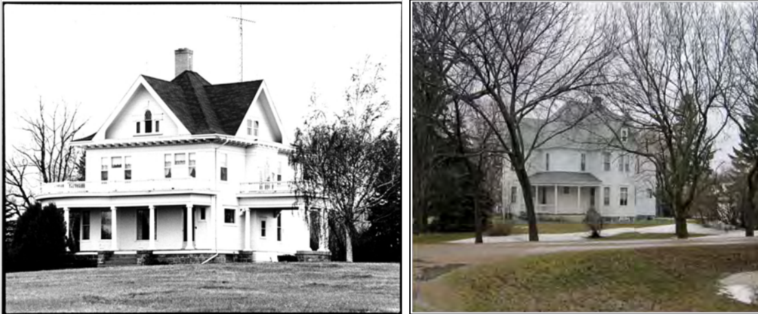
Figure 11. The Ralph Hall Farm Residence and House HDR 26400/42860 The Ralph Hall Farm residence in Carrington (on left) is similar in style to the house recorded at HDR 26400/42860 (on right) in Ora Township within Nelson County.
