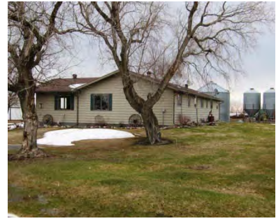
Ranch residence to northwest of barn view to south.
