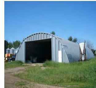
Modern metal Quonset building HDR 11932/41403 Rosefield Township, Eddy County
