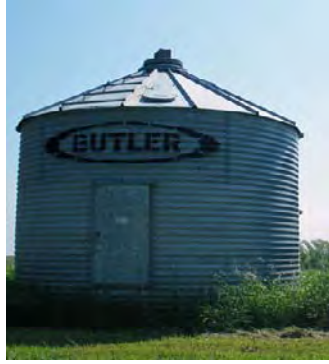
Butler grain bin HDR 26389/41731 Ora Township, Nelson County
