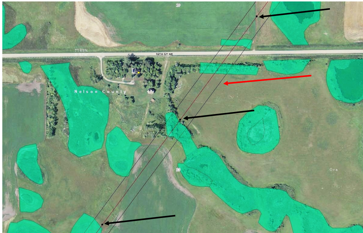
Figure 4 View to north of subject property. Red arrow depicts location of proposed Minnkota transmission lines. Black arrows show location of proposed single-pole structures.
