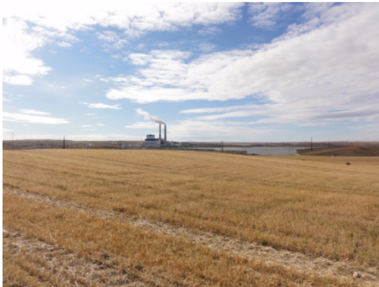
Photo 1: Site CGF-A-1, View to Southwest
