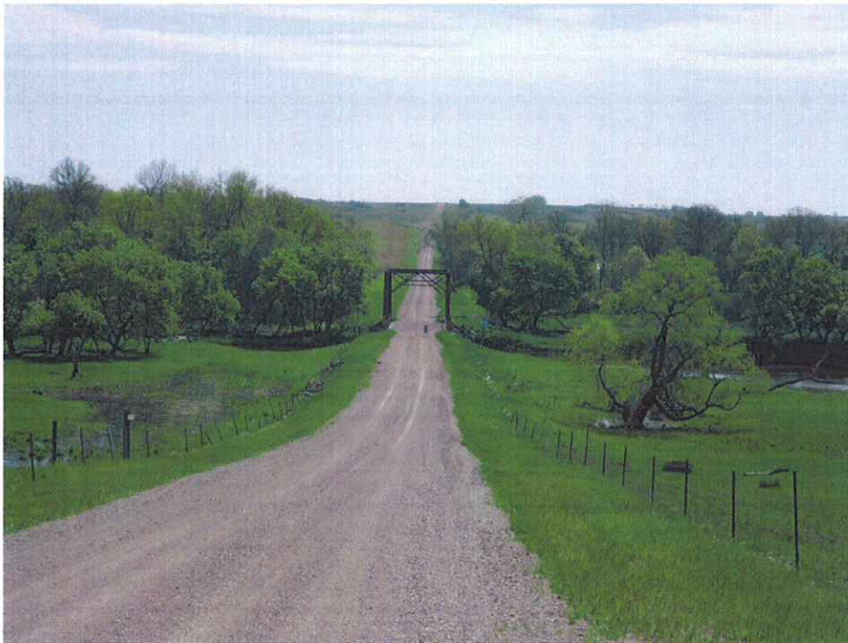
Photo 4 – Sheyenne River Crossing
