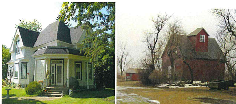
Figures 2-3 Queen Anne style residence and granary at the subject property
