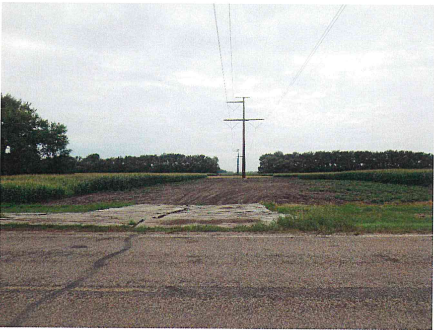
Photo 4: Pole 753, showing construction matting, looking east.
