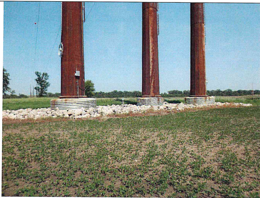
Photo 1: Pole 69 base, looking east across the Missouri River.
