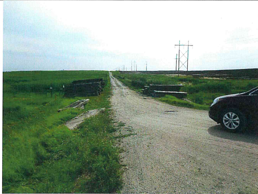
Photo 3: Pole 256 showing construction matting, looking east.
