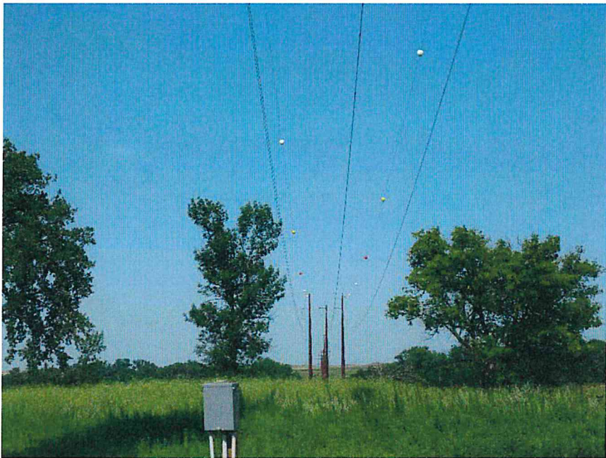
Photo 2: Pole 70, looking east across Missouri River.
