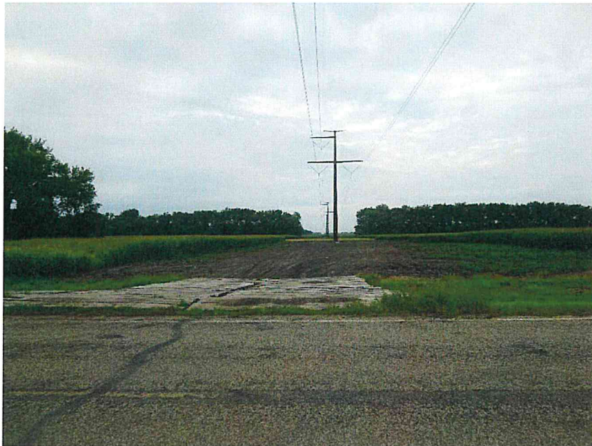
Photo 4: Pole 753, showing construction matting, looking east.
